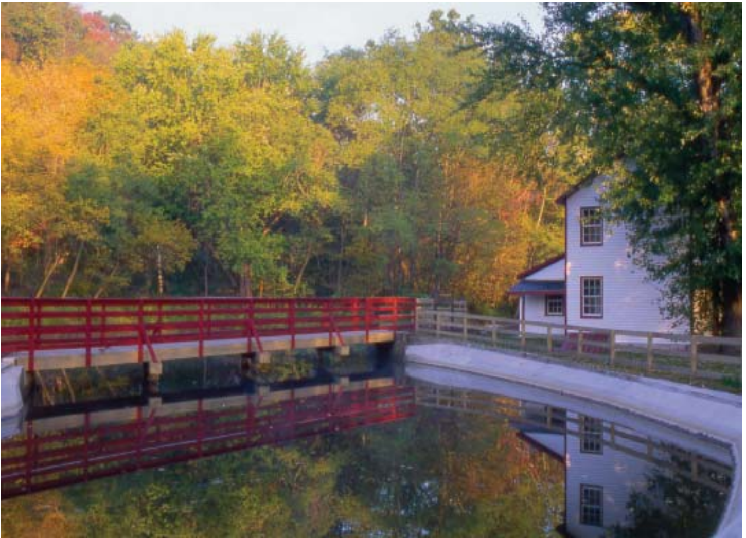
Restored features enhance Delaware Canal State Park.
