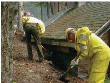
Removing pine needles and leaf litter from the roof and around the house is a Firewise practice.
