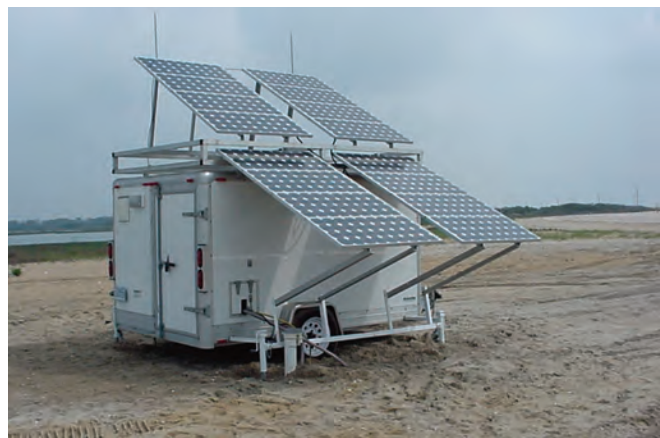
Photovoltaic panels on a trailer power the pump that brings water to the showers. Note the pvc pipe coming out of the ground to the left of the wheel. The power is carried by cable down the pipe to the pump in the well. NPS photo.
