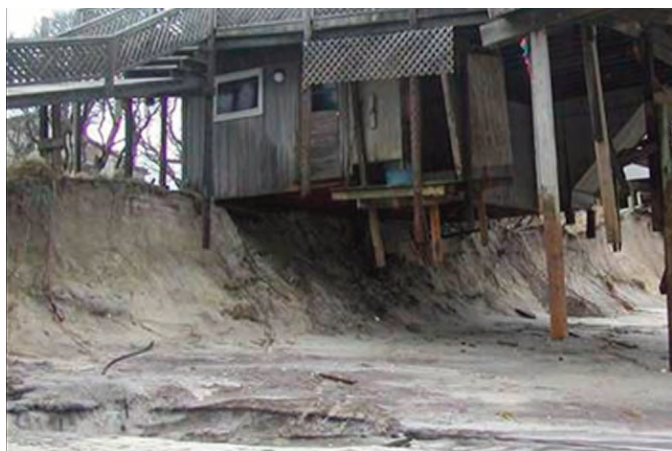
Figure 1. Structural damage caused by shoreline erosion in the community of Davis Park at Fire Island National Seashore. NPS photo.
