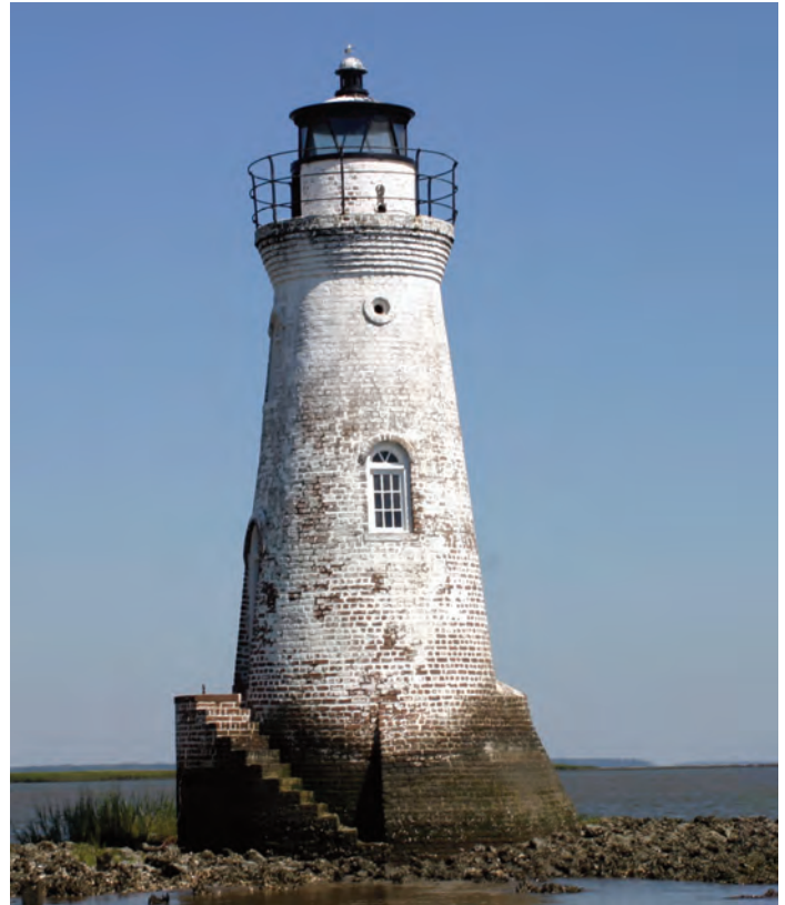
The Cockspur Lighthouse at Fort Pulaski NM demonstrates the need for adaptation strategies to respond to the rising sea. Notice the high water line at the base of the lighthouse. Current projections indicate sea level in this area may rise as much as 2.3 feet over the next 50 years. NPS photo.
