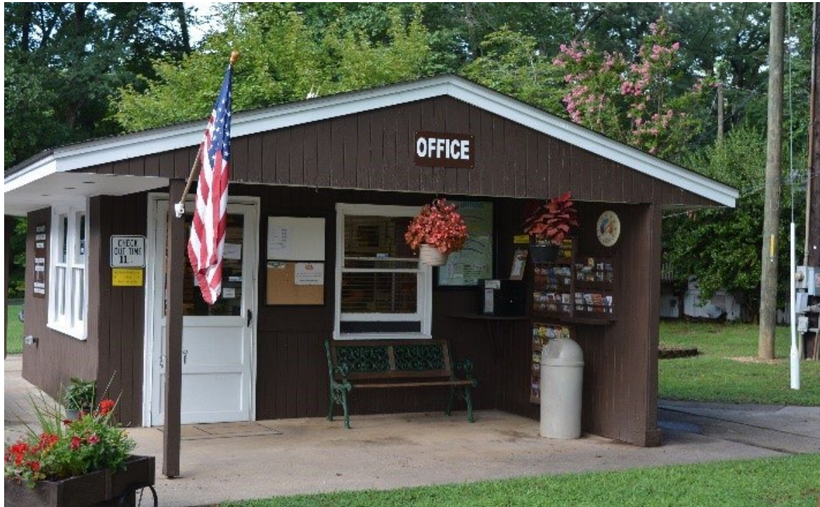
Pictured: Prince William Forest Park RV Campground Office
