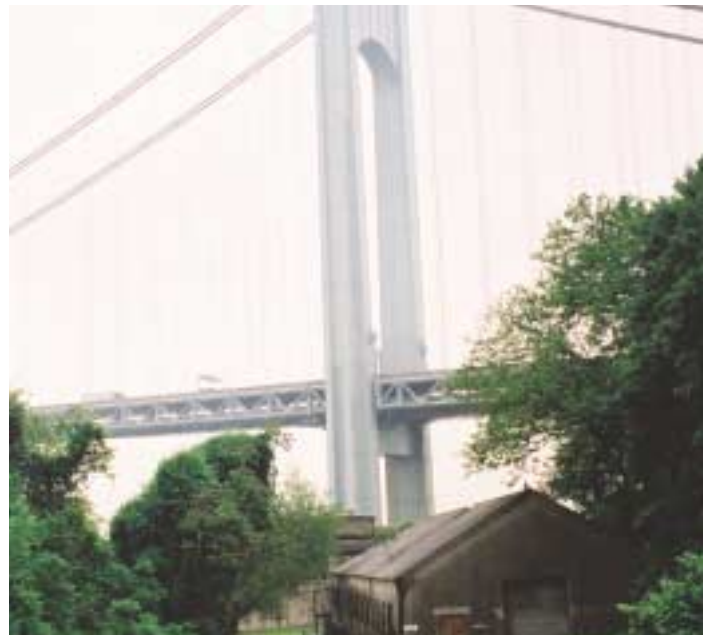
Teleconferencing between the Jamaica Bay and Staten Island units could reduce VMT over the Verrazano Bridge, as seen above from Fort Wadsworth.
