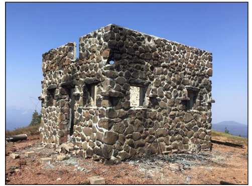
The Dixie Fire destroyed wooden portions of the historic Mr. Harkness Fire Lookout in Lassen Volcanic National Park. NPS Photo
