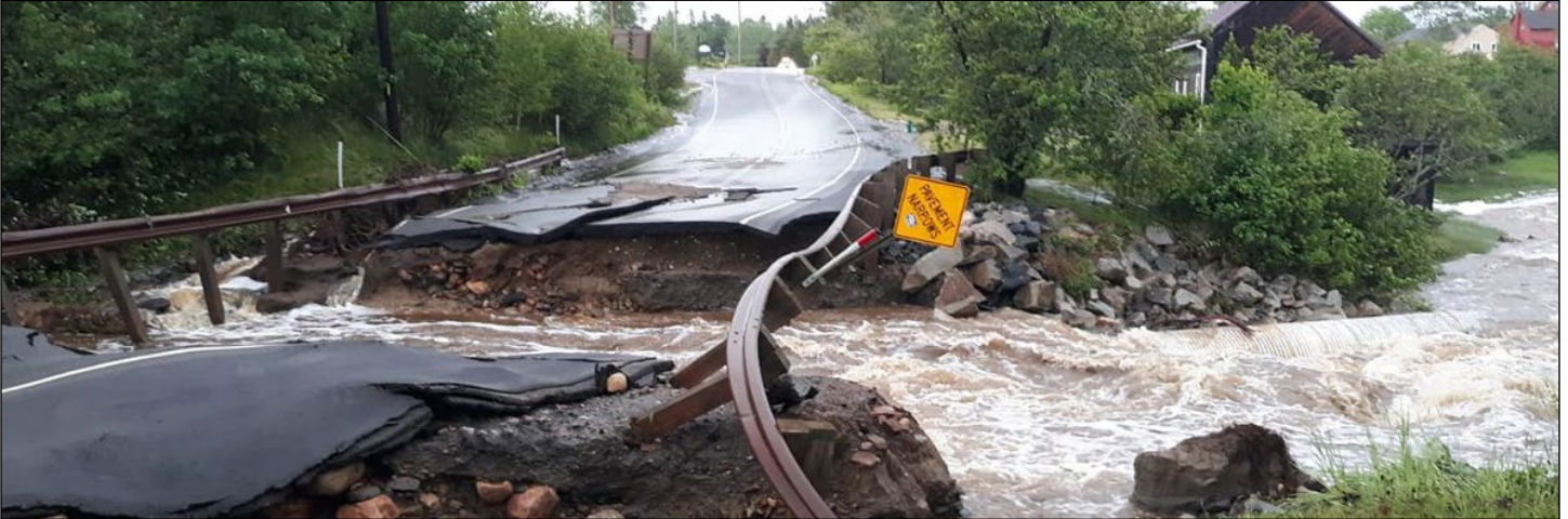
A bridge on Route 186—a major access point for the Schoodic Institute at Acadia National Park—collapsed as a result of torrential rainfall in June 2021. Photo by Natasha Foutch.
