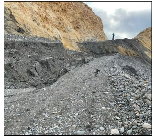
A displacement of approximately 14 vertical feet occurred over two weeks at Pretty Rocks Landslide in Denali National Park in 2021. NPS Photo
