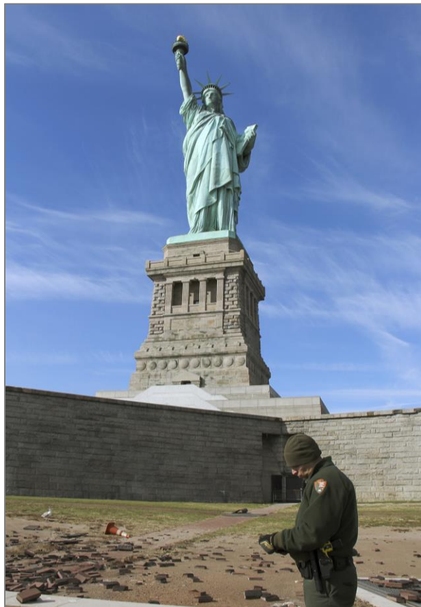
Photo 3. A National Park Service ranger surveys damage from the aftermath of Hurricane Sandy at Statue of Liberty National Monument, NY. Photo credit: National Park Service.
