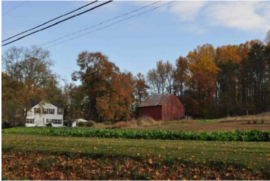
A well sited rural home adjacent to cropland in Prince George's County
