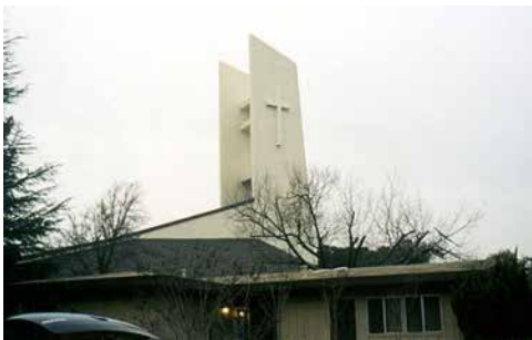
Examples of disguising cell towers: Cemetery, flagpole, and church steeple
