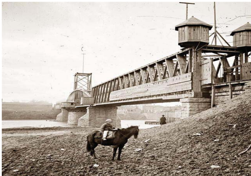
Blockhouses protecting the railroad over the Cumberland River at Nashville, Tennessee
