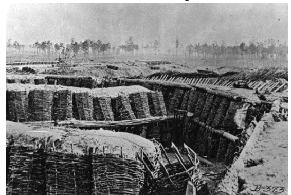
Use of gabions and fascines
