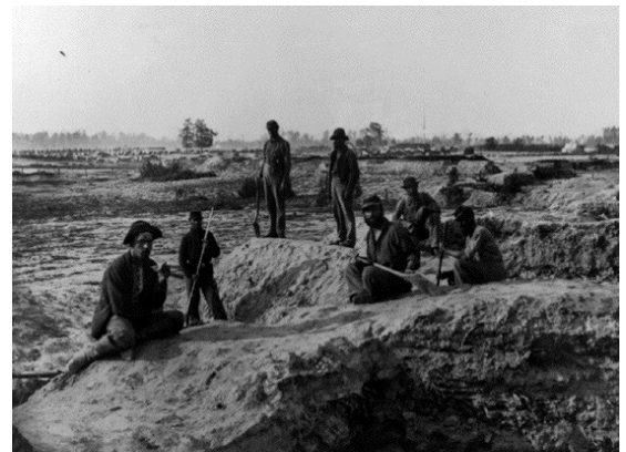
Soldiers constructing earthworks during the war
