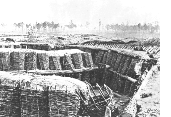
Use of gabions and fascines
