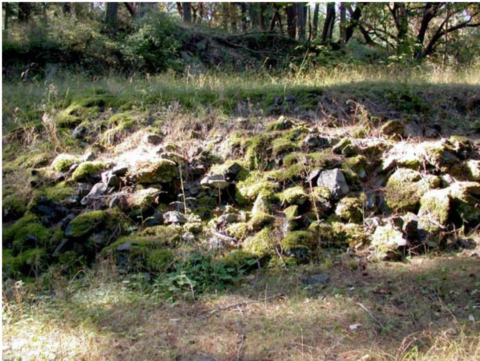
Contemporary photo of a retaining wall on the top terrace of Officers' Hill. (CCSO, 2003)
