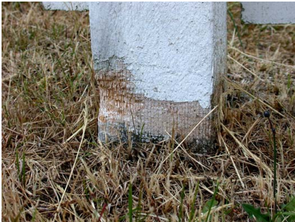
Contemporary photo of one of the fence posts in the parade ground fence at American Camp. Many of the fence posts have been damaged by lawn care practices. (CCSO, 2003)
