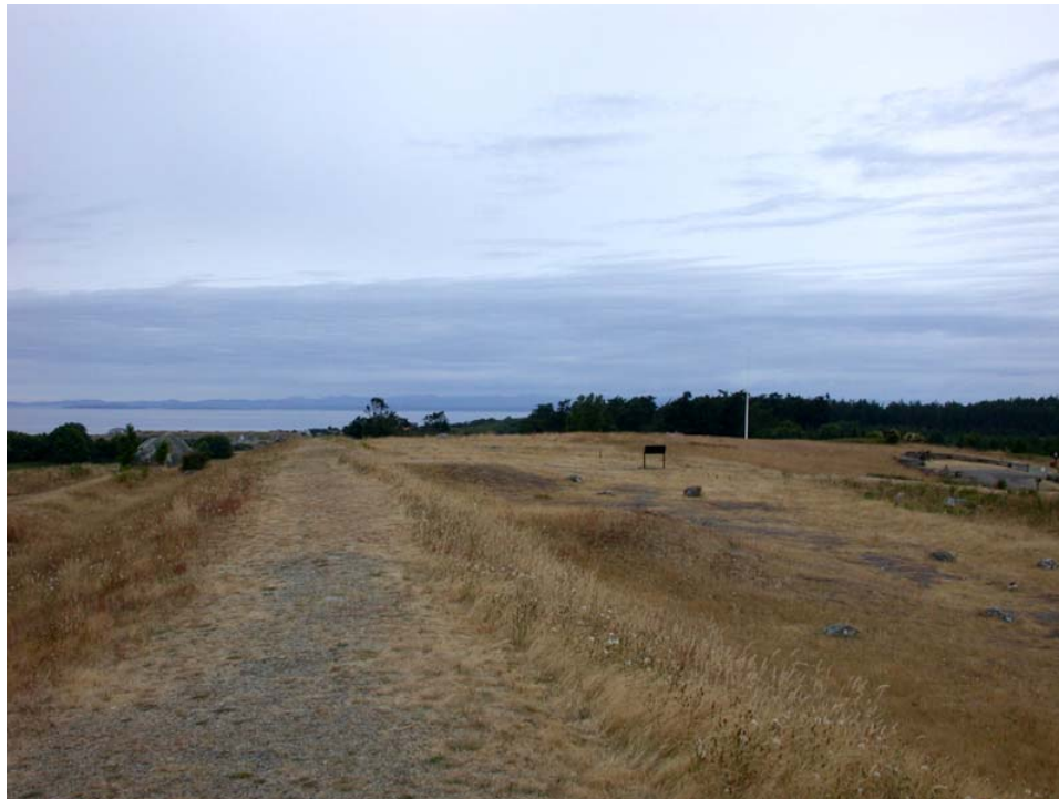
Contemporary view of the redoubt. Visible in the photo is the south side of the main fortifications with two of the gun platforms. (CCSO, 2003)
