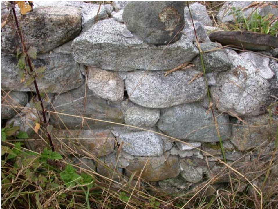
Contemporary photo of a mortared stone and brick foundation near an orchard remnant. This may have been from an early homestead structure, and probably postdates the military period. (CCSO, 2003)
