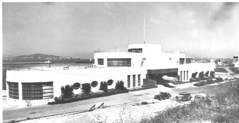
Figure 117. View of the Bathhouse from the hill north of Beach Street, showing the vegetation and character of plantings across the front façade of the building. View looking northeast, ca. 1940. ( San Francisco Maritime NHP, Historic Documents, Photograph Collection, P81-073,2n )
