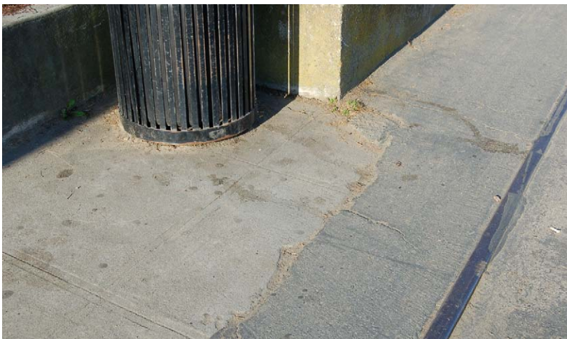
Figure 100. In some areas walkways have been resurfaced with paving added over existing layers creating a patchwork of materials. (NPS, 2008)
