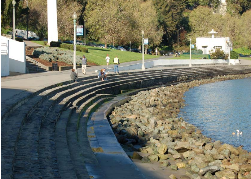
Figure 52. Current view of Seawall around the cove stepping to the Beach Promenade and the slope above to the Upper Promenade. View looking west. (NPS, 2006)
