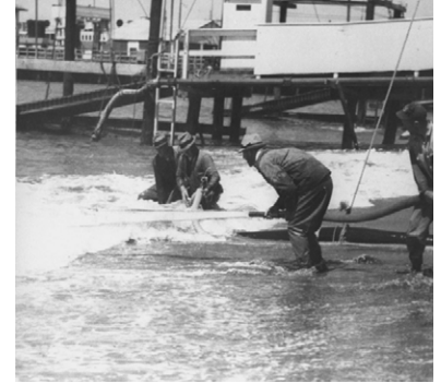
Figure 26. Agitating with hoses to redistribute sand and replenish the beach, 1939. (Courtesy of the San Francisco History Center, San Francisco Public Library, AAA 6708)
