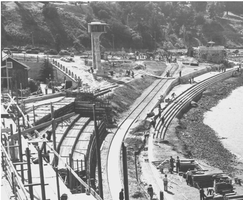
Figure 50. Detail of WPA photograph showing the number of topographic modifications to the slope around the cove that were part of the site design and construction of Aquatic Park, 1938. ( San Francisco Maritime NHP, Historic Documents, Photograph Collection, P88-035.00139 )
