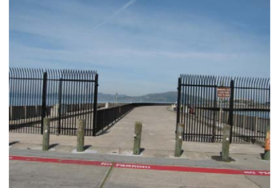
Figure 64. Fencing was added to the Municipal Pier in 2008 and 2009 to enhance safety until structural improvements can be completed. View looking north. (NPS, 2010)
