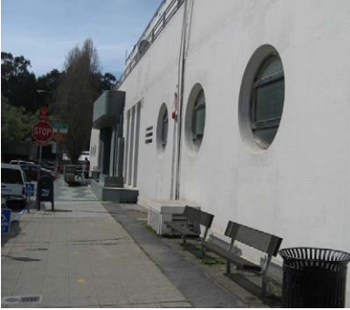
Figure 88. Northeast side of the entrance to the Bathhouse with a variety of non-compatible features such as benches, trash cans, city street signs, utilities, and public mailbox. (NPS, 2010)
