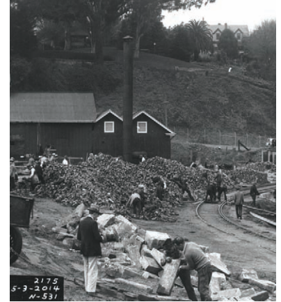
Figure 11. Collected from city improvement projects, a variety of salvage materials were brought to the site and used as fill material. View looking west. ( San Francisco Maritime NHP, Historic Documents, Photograph Collection, P88-035.00027 )
