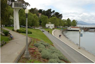
Figure 71. View of three components of the pedestrian circulation system in Aquatic Park. The Beach Promenade along the shoreline, the State Belt Railroad tracks (asphalt), and a portion of the Upper Promenade as it passes the West Speaker Tower. (NPS, 2008)
