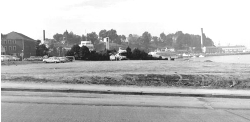
Figure 33. View of Lot 9 and the future Victorian Park east of Aquatic Park, prior to construction of the cable car turnaround. View looking west, 1955 (Courtesy of the San Francisco History Center, San Francisco Public Library, AAA 6742)
