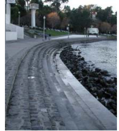
Figure 61. One of the earliest structures built by the WPA, the Seawall wraps around the cove, creating a hard edge between the water and the Beach Promenade. View looking west. (NPS, 2007)
