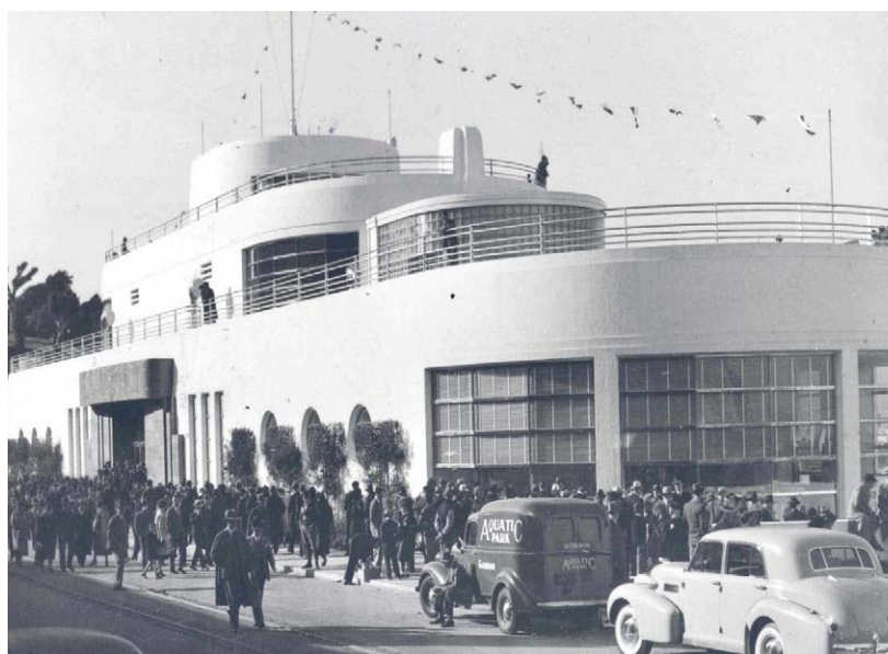
Figure 28. Plantings installed in front of the Bathhouse for Dedication Day, January 22, 1939. View from Beach Street, looking west. ( San Francisco Maritime NHP, Historic Documents, Photograph Collection, P81-073.1n )
