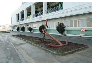
Figure 120. View of the existing juniper plants on the north side of the Bathhouse. View looking south east. (NPS, 2008)
