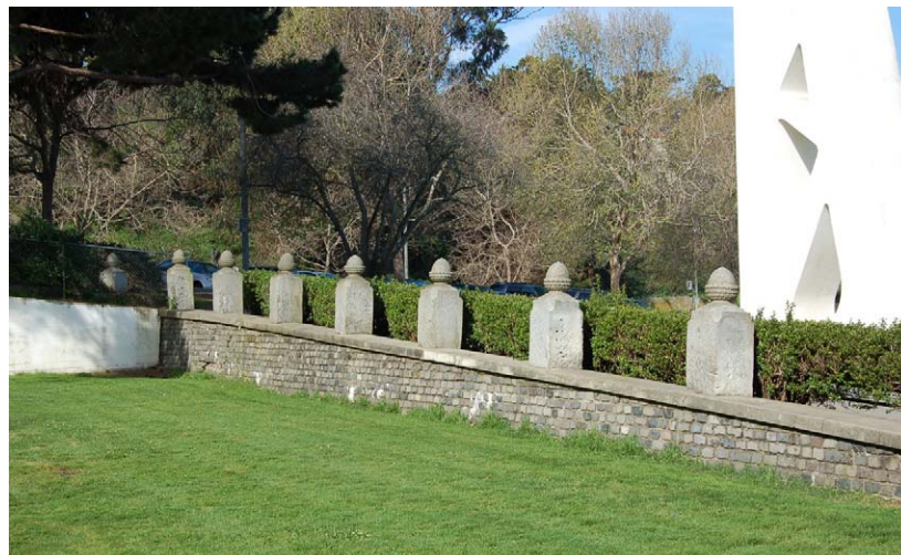
Figure 98. View of the stone retaining wall looking northwest from the lawn near the Bocce Ball Courts. The amount of exposed wall visible in the park today generally slopes to the east based on fill added to even the grade when the pump house was removed in the 1940s. (NPS, 2008)
