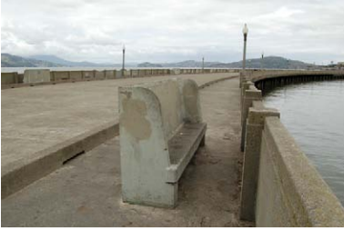
Figure 91. Historic concrete bench, parapet walls and curbing, light standards, and other site features associated with the Municipal Pier. (NPS, 2007)
