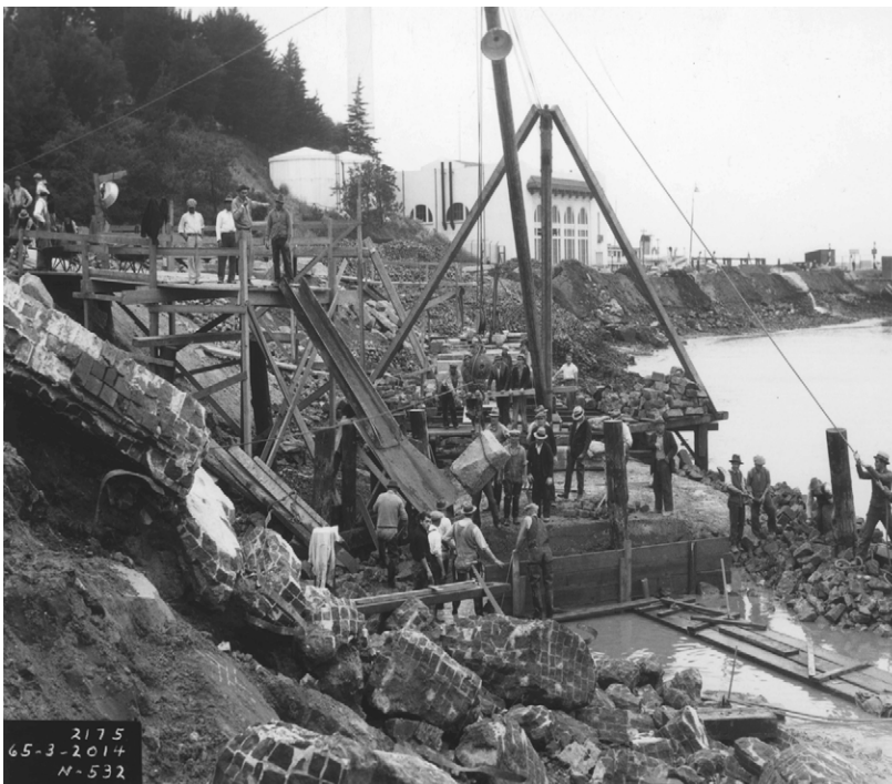
Figure 12. Detail of WPA photograph showing work crews using derricks, pulleys, and other devices to place large stone for the foundations of structures built around the cove. Note the building debris dumped on the slope for use as fill. View looking west. ( San Francisco Maritime NHP, Historic Documents, Photograph Collection, P88-035.00007 )
