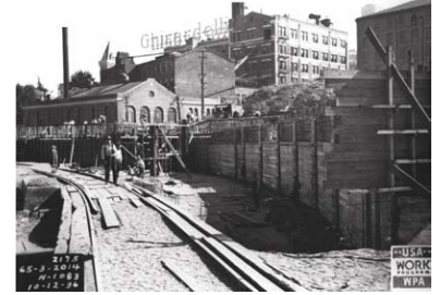
Figure 49. WPA photograph showing the retaining structures required prior to relocation of the State Belt Railroad tracks. ( San Francisco Maritime NHP, Historic Documents, Photograph Collection, SAFR-N-2-26 )
