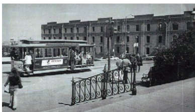
Figure 36. View of Victorian Park and the cable car turn around before the tracks were realigned. ( San Francisco Maritime NHP, Historic Documents, Karl Kortum Collection )
