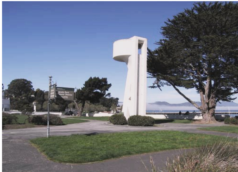
Figure 72. View of the East Speaker Tower and walkways looking northwest from edge of Victorian Park. (NPS, 2007)
