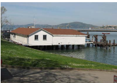
Figure 60. Sea Scout building at the west end of the cove. View looking north (NPS, 2010)
