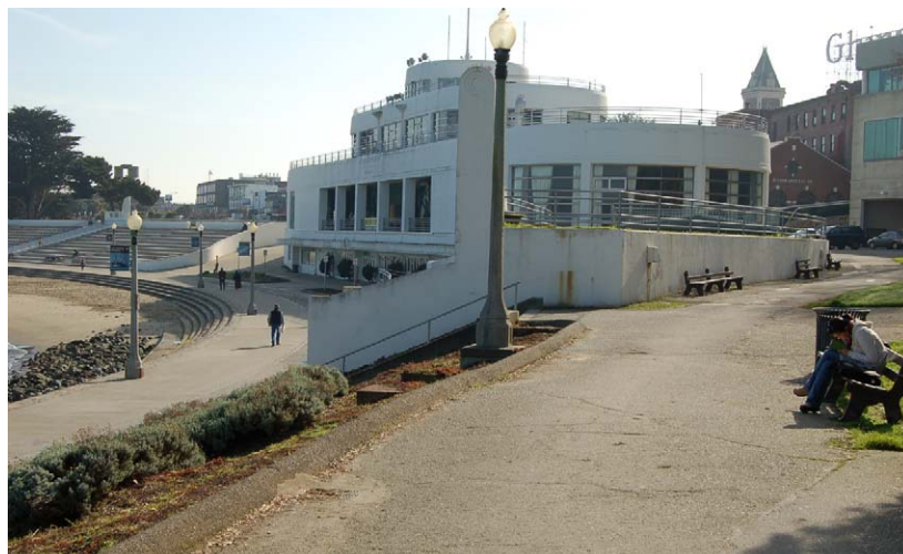
Figure 104. View of the Upper Promenade showing the rolled curb along the edge of the walkway and planting bed (left), and the patching and expansion of paving leaving a relatively undefined edge on the right side. (NPS, 2006)
