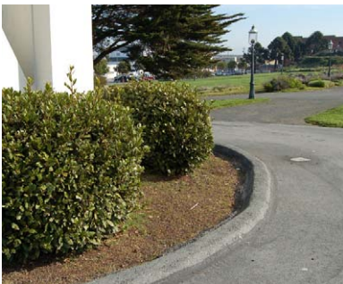
Figure 106. Raised asphalt curb around the East Speaker Tower planting bed. (NPS, 2008)
