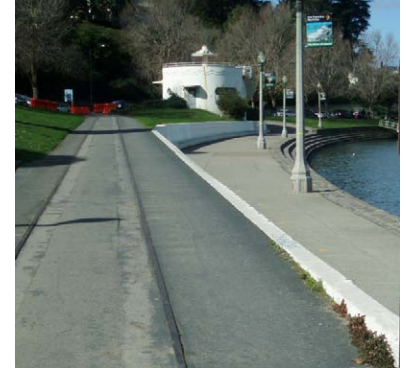
Figure 69. Asphalt walkway located between the Beach Promenade and the slope up to the Upper Promenade with the tracks at grade. (NPS, 2007)
