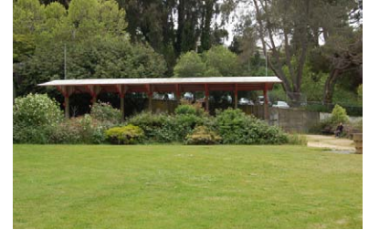
Figure 44. View of the overhead structure covering the Bocce Ball Courts located in the southwest corner of the park. (NPS, 2007)
