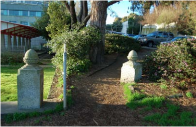
Figure 97. Remnant features of the original stone retaining wall as it wrapped around the park to Van Ness Avenue. View looking south. (NPS, 2008)
