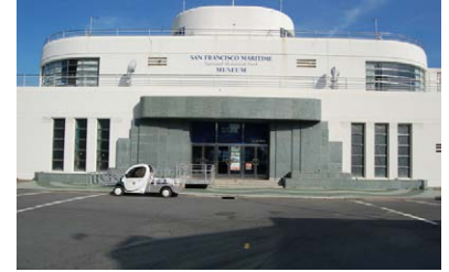
Figure 86. Front façade of the Bathhouse. View looking north. (NPS, 2006)
