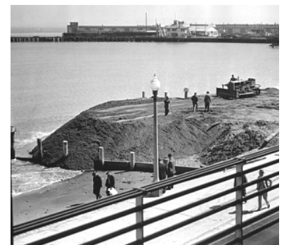
Figure 27. Sand brought to supplement the eroding beach, 1941. View looking east. (Courtesy of the San Francisco History Center, San Francisco Public Library, AAA 6691)
