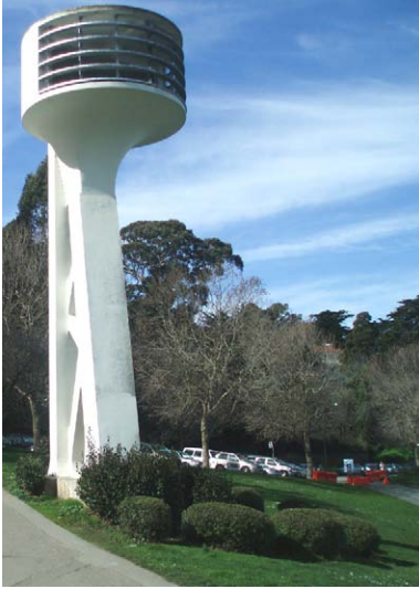
Figure 76. Grecian laurels ( Laurus nobilis ) remaining around the West Speaker Tower. View looking west. (NPS, 2008)
