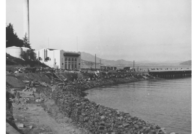
Figure 9. Large amounts of debris and rubble dumped along the shoreline of the cove were used to construct a crude seawall. ( San Francisco Maritime NHP, Historic Documents, Photograph Collection, P88-035.00033 )
