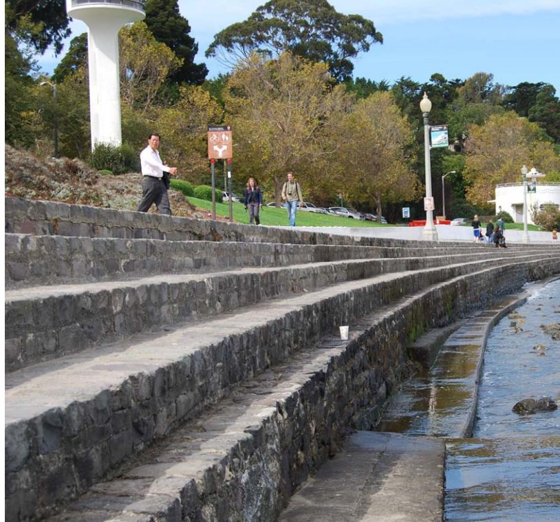
Figure 93. One of the earliest structures built during the historic period, the Seawall around the cove is in relatively stable condition. (NPS, 2009)
