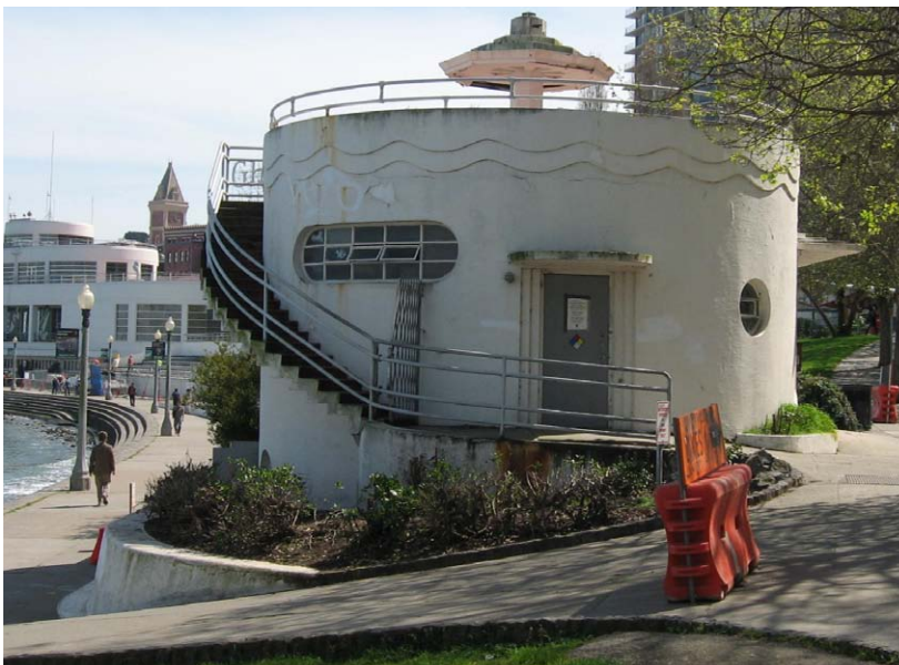
Figure 58. West Convenience Station. View looking east. (NPS 2010)
