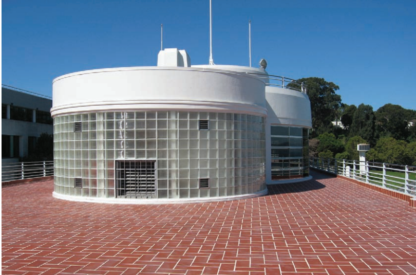
Figure 55. Rehabilitation work at the Bathhouse in 2008 included the installation of a new stainless steel window system; and a modern waterproofing system for the building roofs with new roof tiles to match the historic ones that could not be salvaged. The rehabilitated glass block pantry is now the elevator lobby on the 3rd floor. (NPS, 2008)
