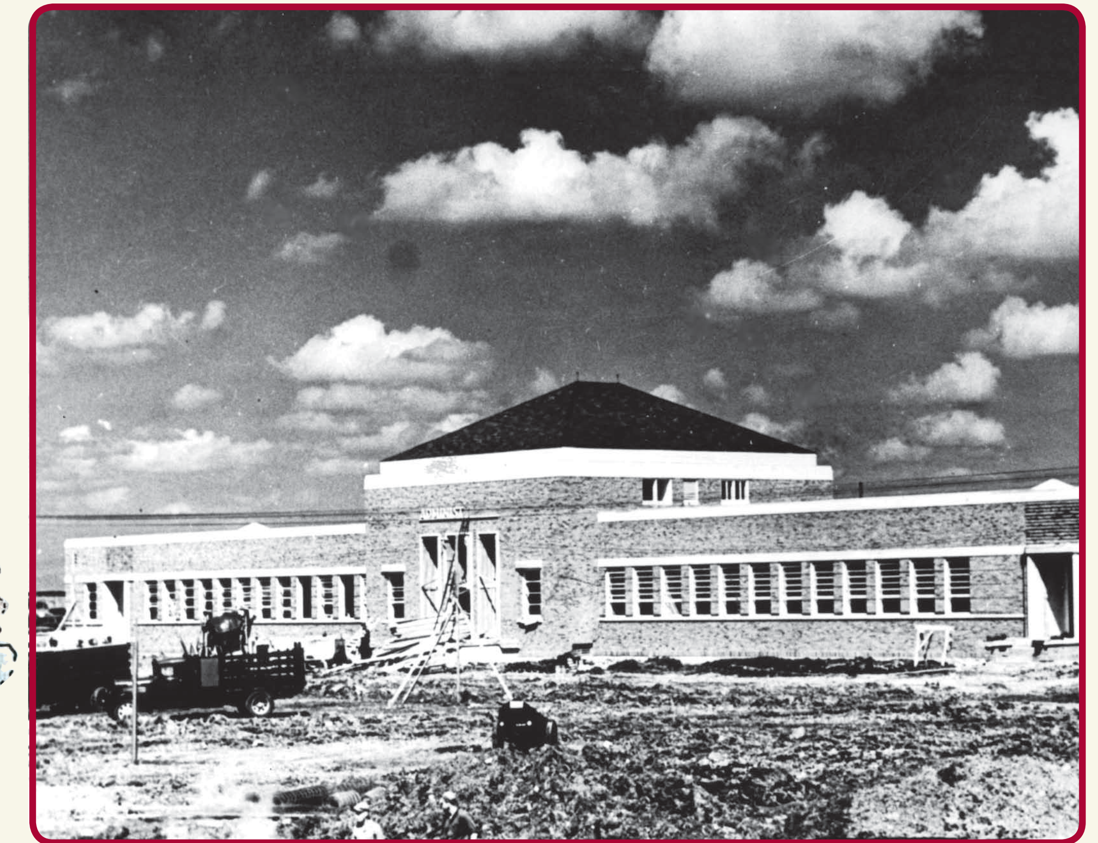
Construction work nears completion on the U.S. Naval Air Station Administration Building in 1942. It was located two miles east of Gardner Junction. Photograph is courtesy of the former Olathe Naval Air Museum and the Johnson County Museum.
