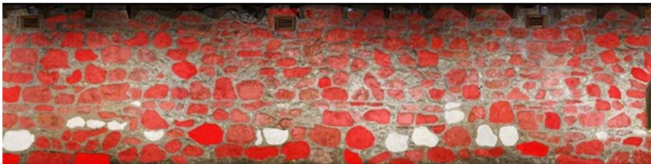
Figure 1.5: Elevation photo with stone thicknesses indicated by different intensities of red. (Author 2019)
