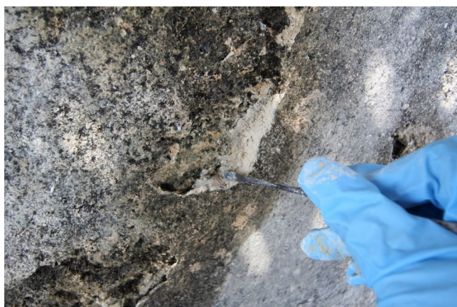
Figure 0.7: Detail of edging mortar applied to the border of fragile plaster remnant as a remedial conservation treatment.
