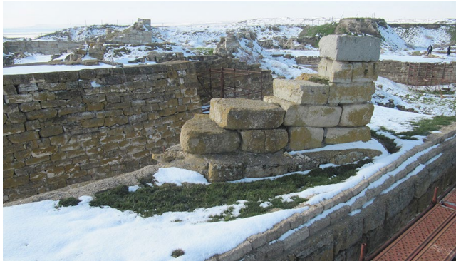
Figure 4.4: In Gordion, Turkey, adobes edged the soil cap which became part of the soil cover. (Photo by Author)
