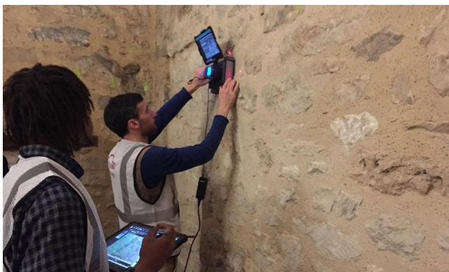
Figure 1.4: View of engineer measuring an individual stone thickness using the Proceq GPR Live unit. (Author 2019)
