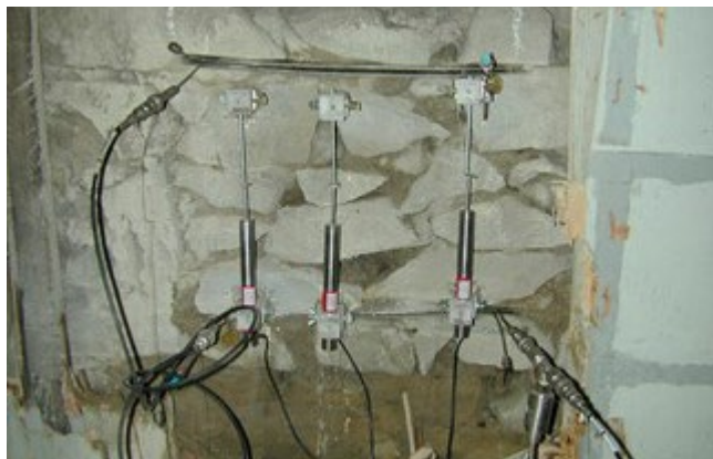
Figure 1.12: In situ compression testing of stone masonry using flatjacks in accordance with ASTM C1197. (Author 2007)
