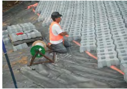
Figure 4 – Articulated Concrete Blocks
