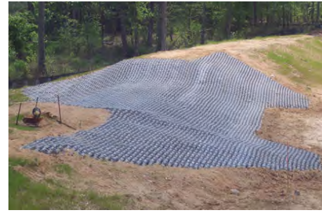
Figure 5 – Example of ACB mat in place
