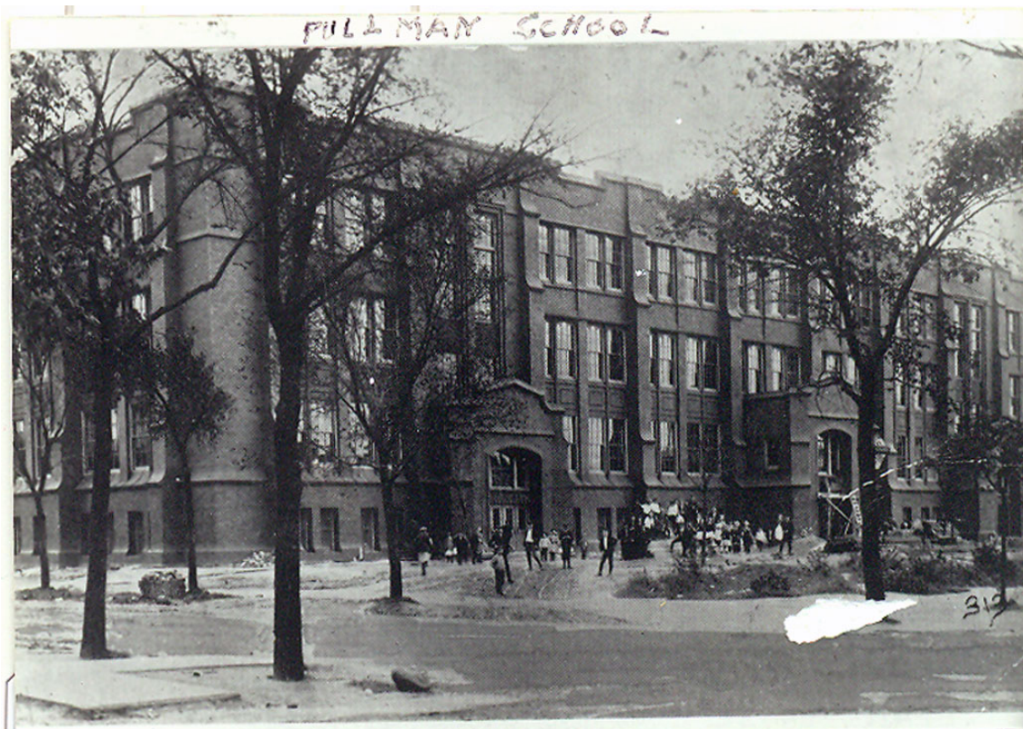
Figure 4.18. Second Pullman School, c. 1910, Perkins & Will, architects. Collection of the Pullman State Historic Site, http://www.pullman-museum.org/main/pfp.11.01.08.21.jpg
