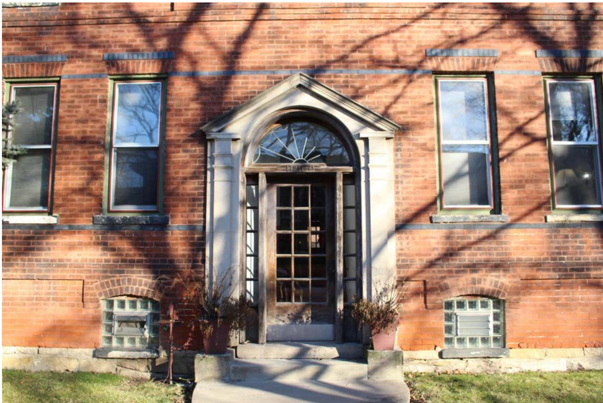
Figure 4.39. Colonial Revival-style door surround added to 11211–13 Champlain Avenue. Photo S. Scarlett.
