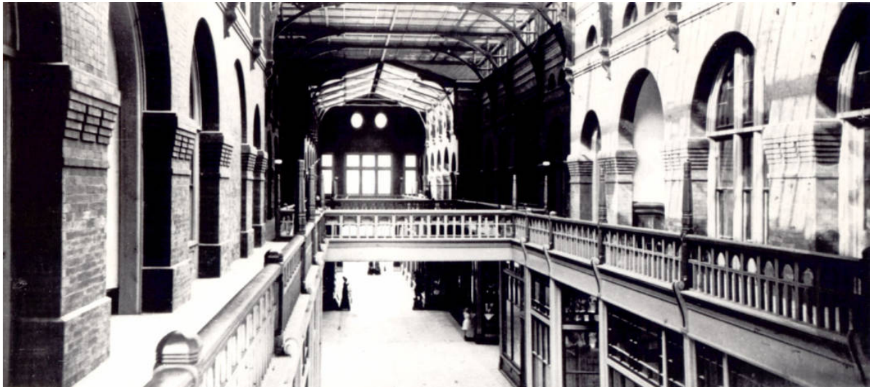
Figure 4.7. Interior of the Arcade showing masonry construction and steel and glass atrium span. The Pullman State Historic Site. Collection: Industrial Heritage Archives - Pullman State Historic Site. Arcade Building Interior" The Pullman State Historic Site Collections. Accessed 2019-08-23. http://www.pullman-museum.org/pshs/pshsFullRecord.php?collection=pshs&pointer=14193
