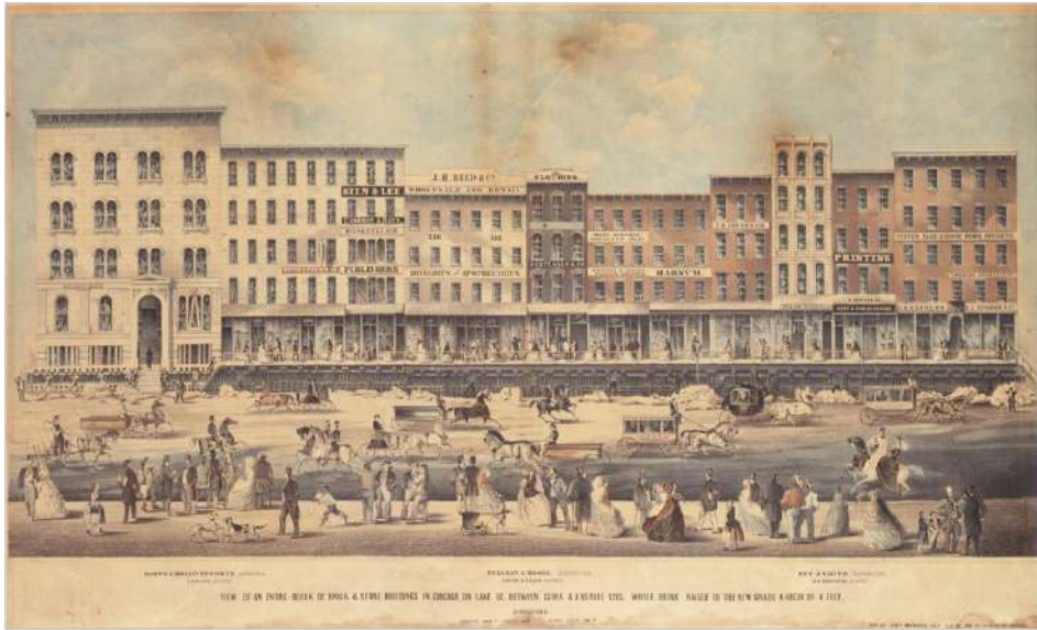
Figure 2.16. “View of an Entire Block of Brick & Stone Buildings in Chicago, on Lake St. Between Clark & LaSalle Strs. While Being Raised to the New Grade a Height of 4 Feet,” by Edward Mendel 1857, Chicago Historical Society.
