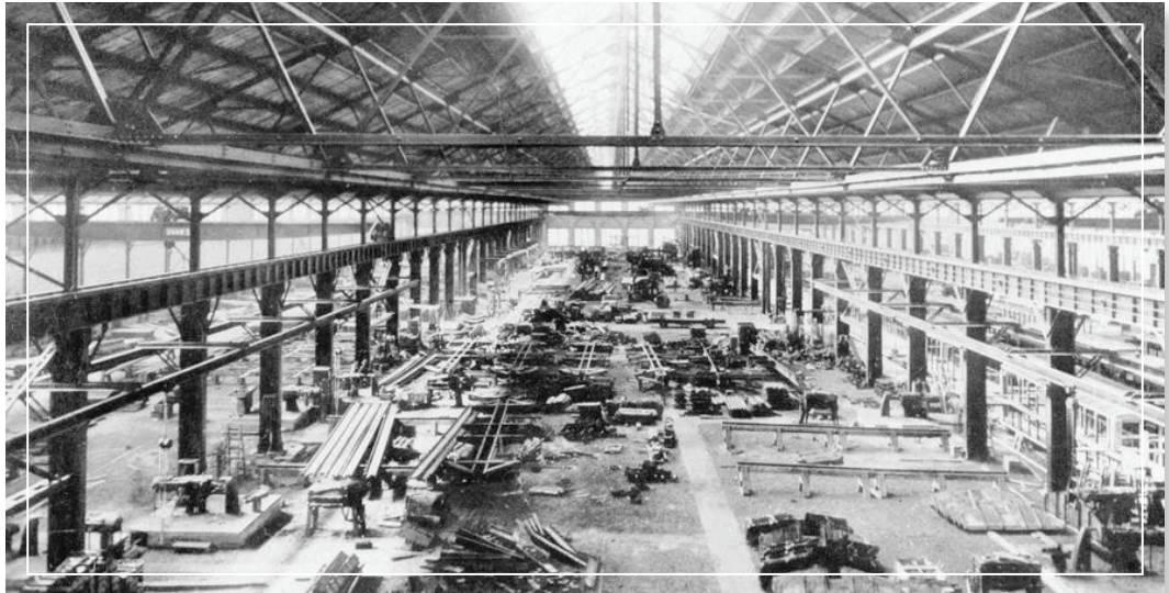
Interior of the Machine Bay, Pullman. Photo: Historic American Engineering Record, Library of Congress, undated photograph.
