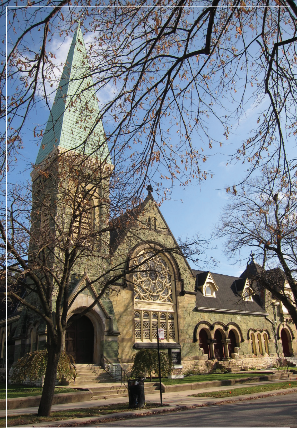
Greenstone Church. 2012. NPS Photo.
