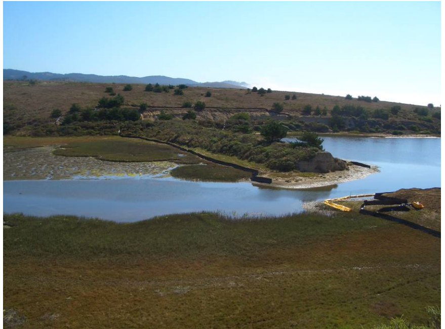
Lower Glenbrook Dam prior to removal of east arm
