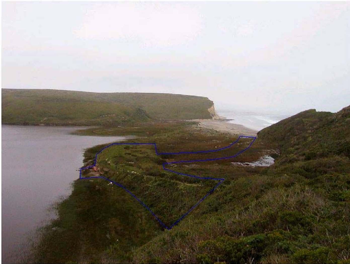
Figure 8. Photo of historic channel site with approximate area of earthen berm to be removed and channel to be established outlined in blue.
