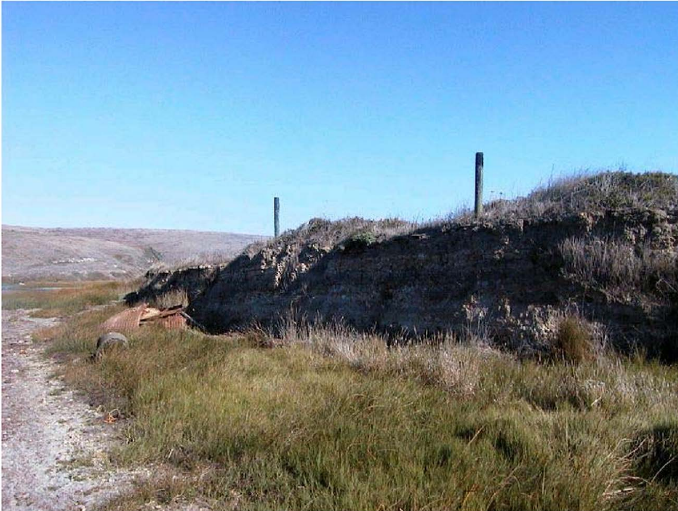
Figure 17. Photo of fill material currently blocking the historic outflow of Horseshoe Pond.
