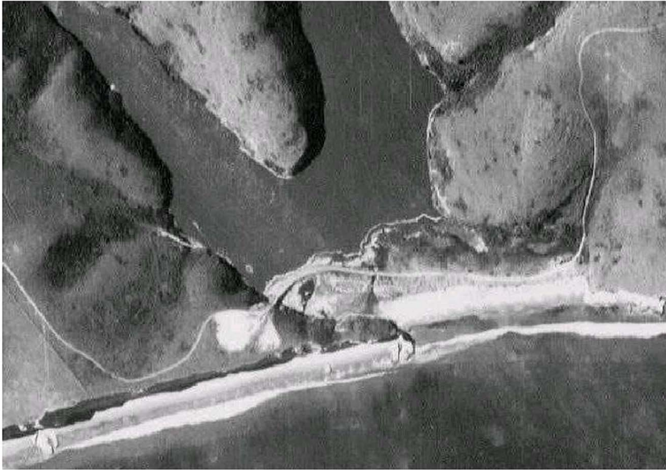
Figure 3. Newly completed road and dam at southern end of Horseshoe Pond. June 6, 1952.
