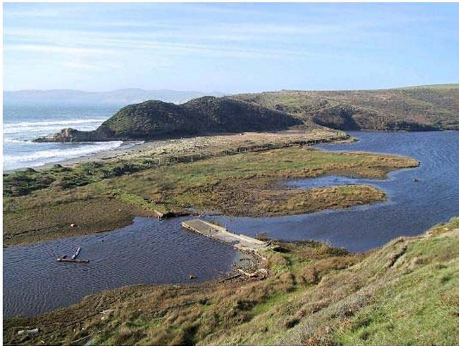
Figures 10 and 11. Photos before and after partial failure of spillway facility showing dramatic loss of water capacity in Horseshoe Pond.
