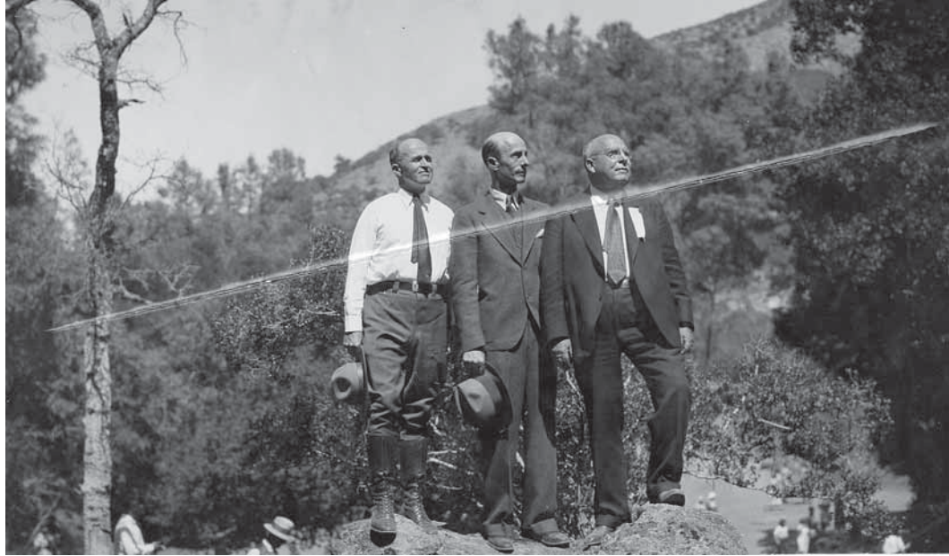
Figure 22. The men principally responsible for the new entrance road, posing on groundbreaking day, October 20, 1932. From left to right: NPS Chief Engineer Kittredge, Col. Goff Thompson, and Custodian W.I. Hawkins. [Mus. Coll. PINN 4372, PNM.]
