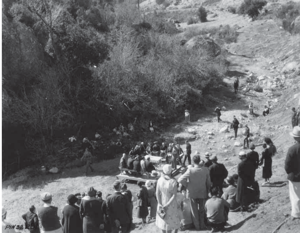
Figure 23. Formal ceremonies on groundbreaking day for the new entrance road, October 20, 1932. The pavillion was located on the lower end of the natural terrace just below the present superintendent's residence (Building #19). [Mus. Coll. PINN 4372, PNM.]
