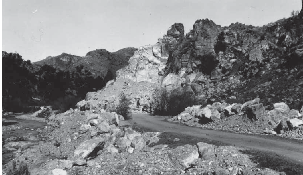
Figure 40. Old Pinnacles Road being constructed above the CCC camp. Exposed rock in background is the quarry, where material for many other projects throughout the monument was taken. [Landscape Architects' Reports, PINN Coll. 3658, Misc. Boxes, PNM.]
