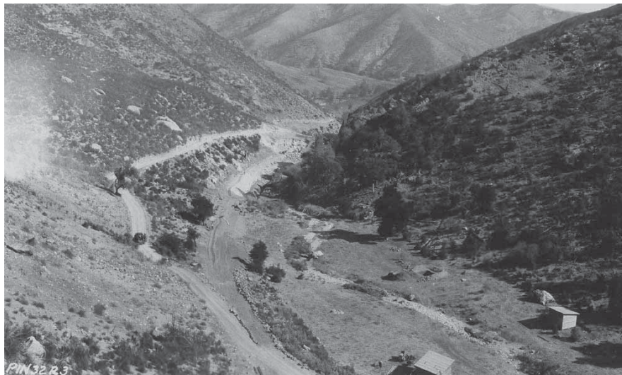
Figure 25. View from above looking east down Bear Gulch in early 1933. Original 1925 road is still extant to left. New road in progress below it. The buildings to the right are the blacksmith's shop and powder room. They were removed shortly after the project was completed. [Included in E.A. Kittredge, "Final Report on Construction of Entrance Road," April 15, 1933, Mus. Coll. PINN 3658, PNM.]
