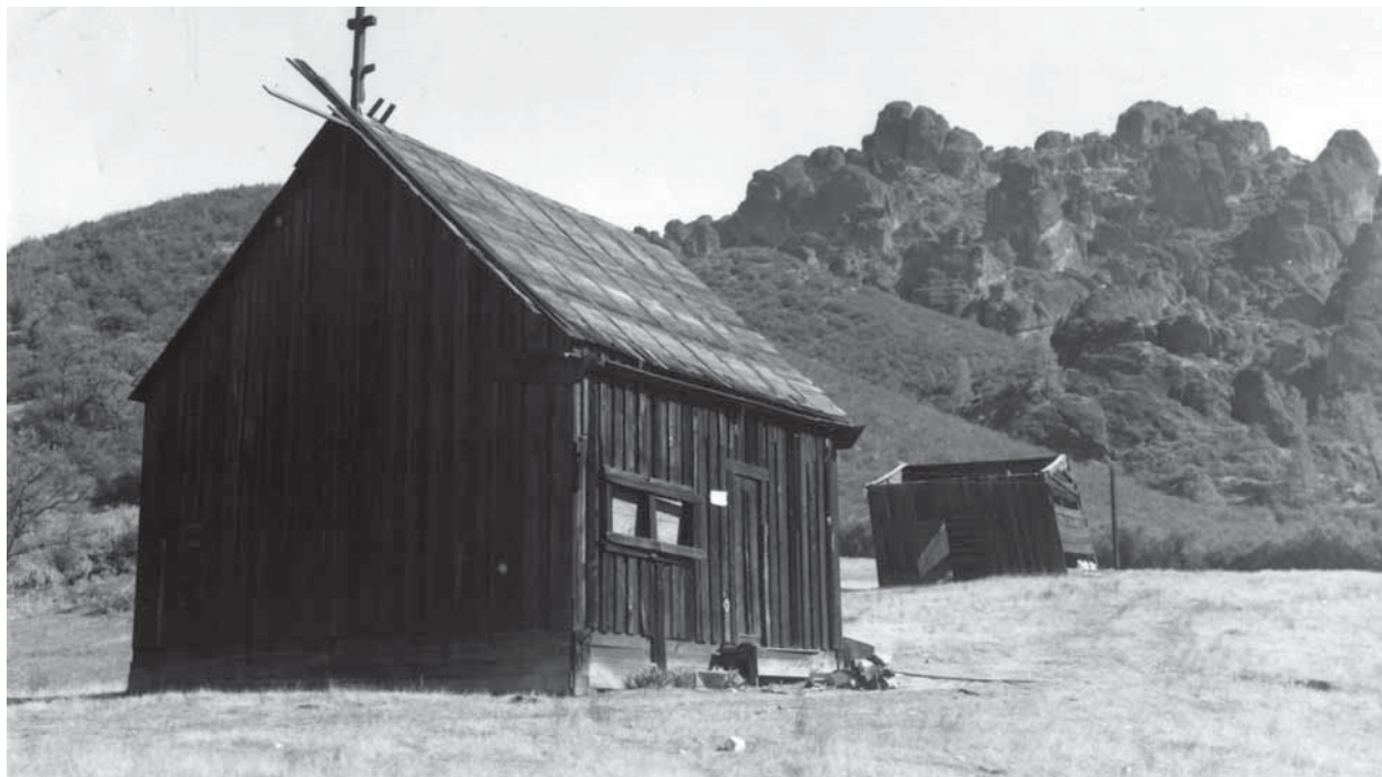
Figure 6. Henry Melville's cabin on the west side of Pinnacles, where Ernest Bauman and later Olive Rivers resided. This photo was taken in the late thirties or early forties, not long before the structures were torn down. They had been abandoned for at least five years by then. [Mus. Coll. PINN 4372, PNM.]
