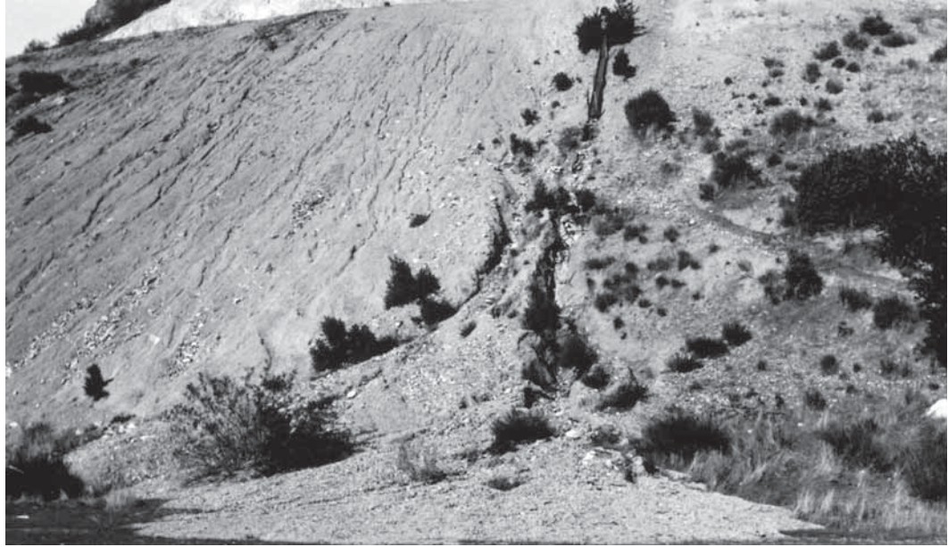
Figure 42. Erosion into Chalone Creek from Bear Gulch Entrance Road a few years after its completion. [Landscape Architects' Reports, PINN Coll. 3658, Misc. Boxes, PNM.]
