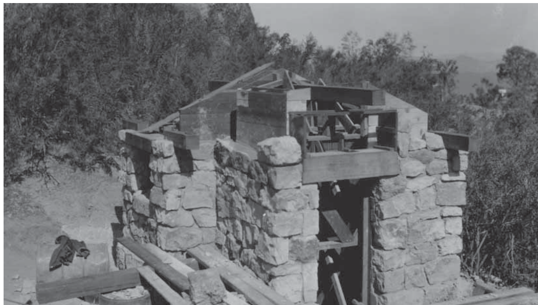
Figure 38. CCC enrollees in process of constructing rustic vault toilet at Scout Peak on the High Peaks trail. [Narrative Reports, CCC Coll., RG 35, Box 22, NARA II.]
