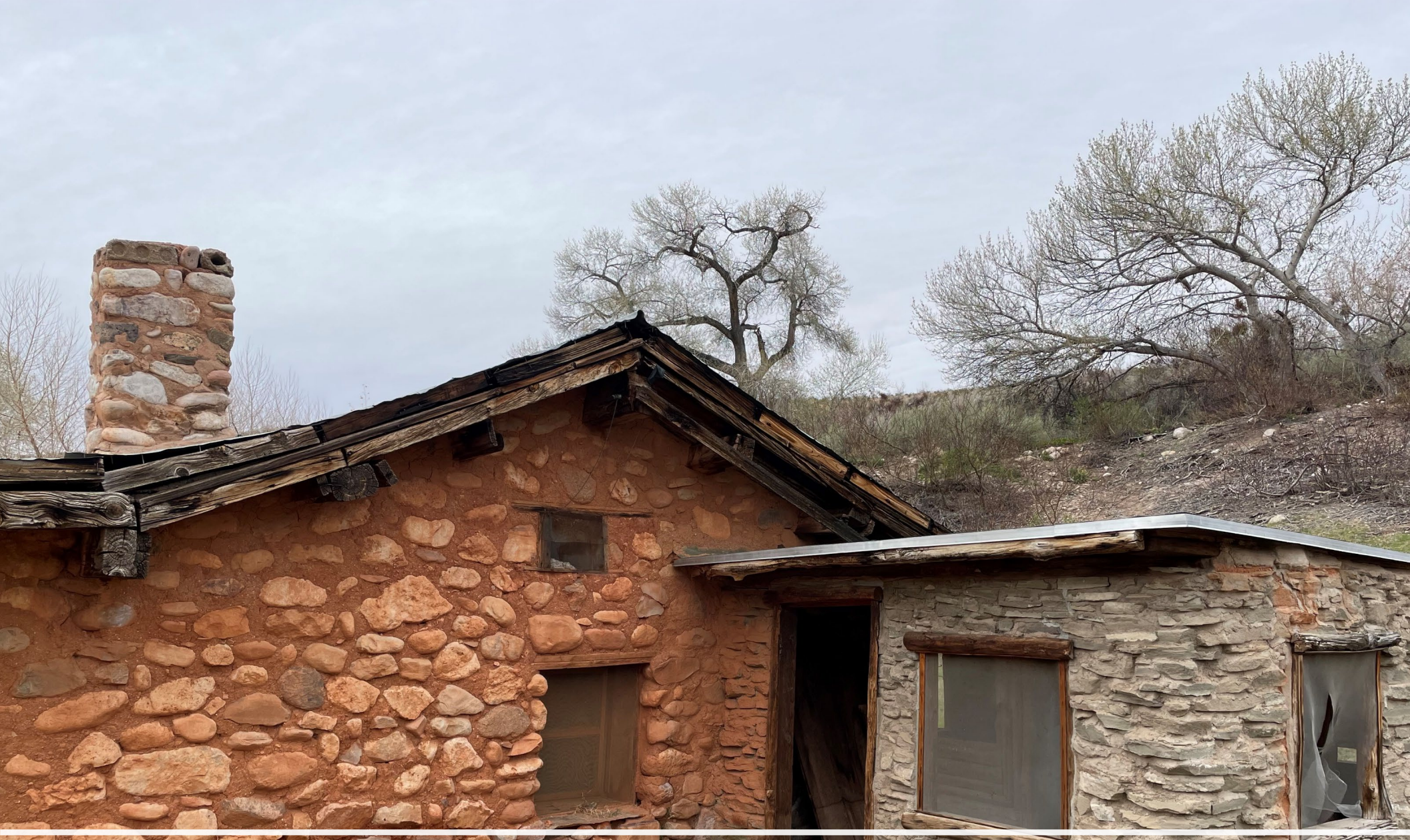
Tassi Ranch: Tucked in rocky hills beside a flowing spring, a rustic stone house and other ramshackle structures paint a vivid picture of life on a cattle ranch in the 1930s and 1940s.
