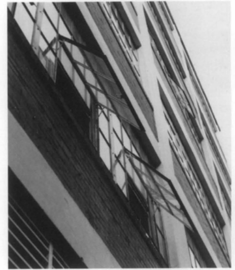
Figure 7. Retrofitting projecting ventilator with the TRUTH hinges. Photo: Robert Powers.
