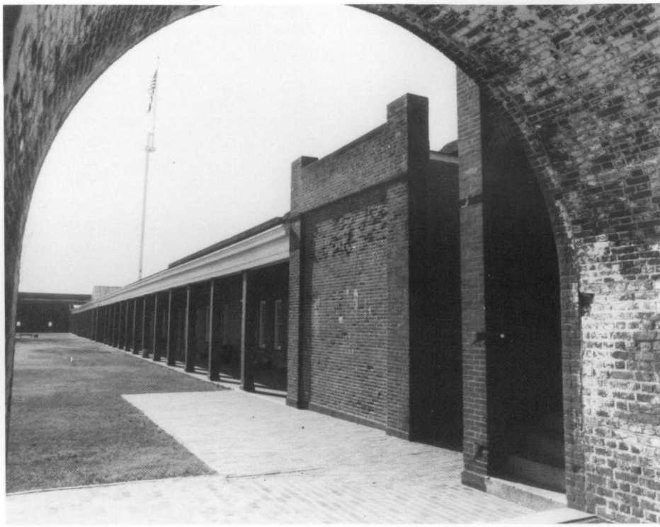
Figure 2. View from one of the open casemates, looking across a portion of the parade ground. The piazza provides a covered access to the enclosed casemates which flank the sally port. It was one of these enclosed casemates (each has a door and one or two windows) that was selected to house the museum object storage facility.
