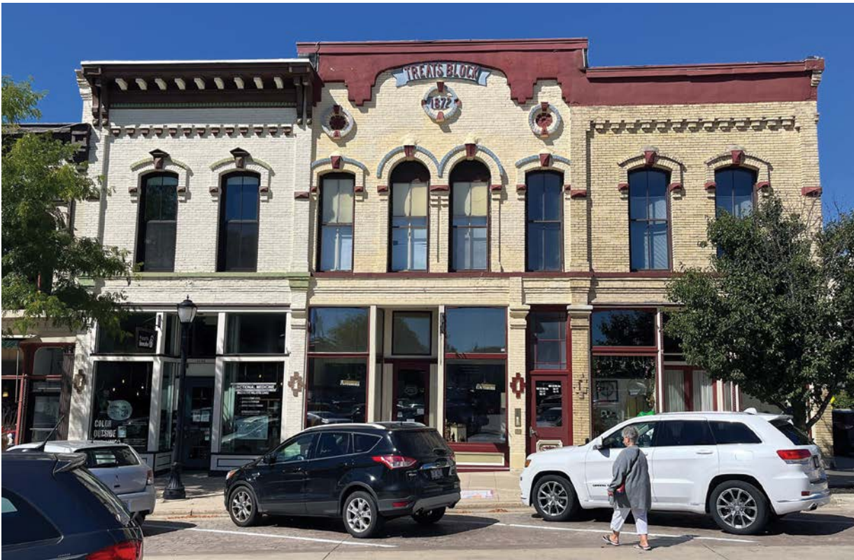
Figure 18. The building code review for this mixed-use building in Monroe, WI, included a comparison of requirements established by application of the three compliance Methods of the IEBC. In lieu of a sprinkler system, the Performance Compliance Method permitted the use of other fire and life safety features. Photo: Chris Rute
