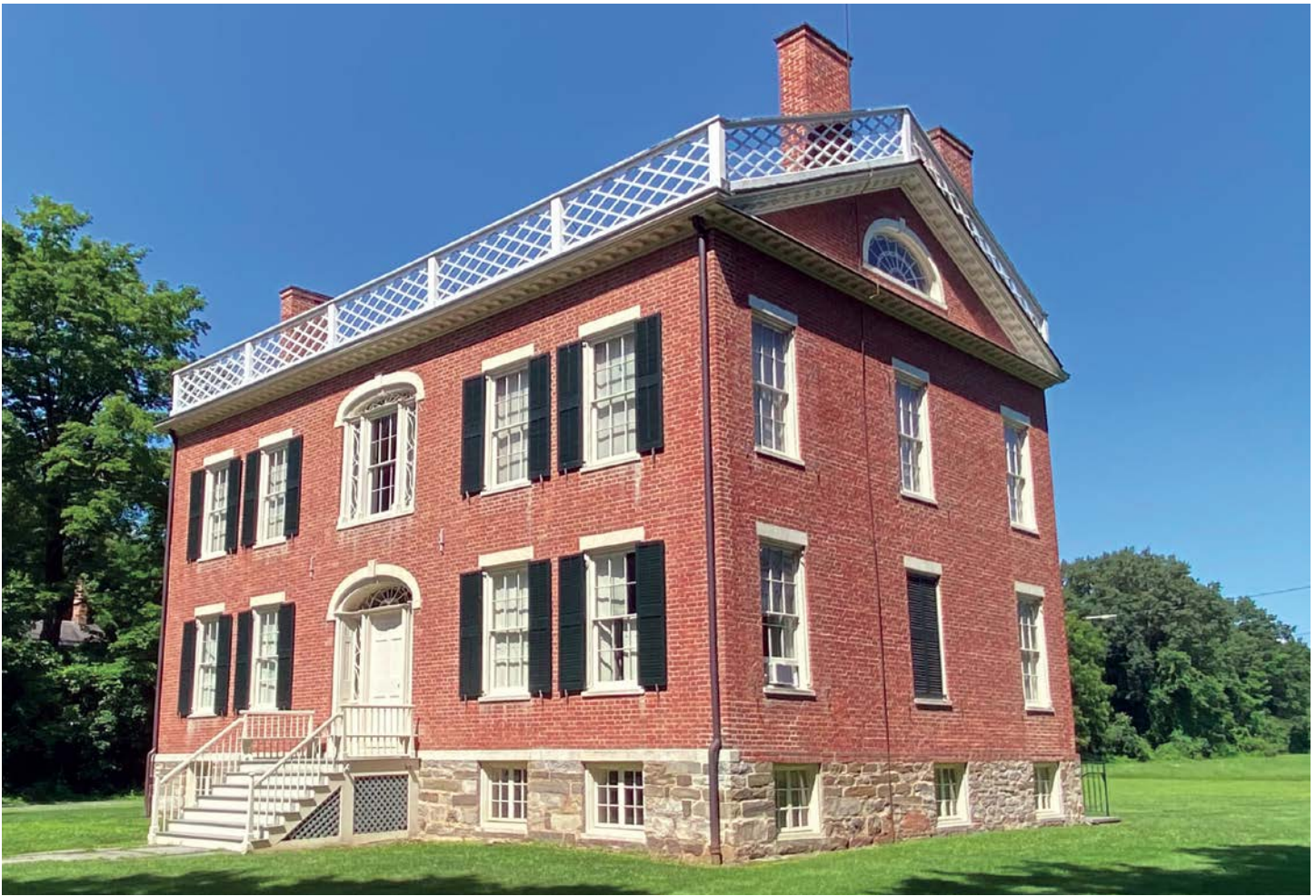
Figure 15. Small and mid-size house museums are provided special treatment in the IEBC, provided that adequate exiting is available. Given the level of careful oversight of these buildings, house museums can be great candidates to use the alternate approaches contained in NFPA 914. Photo: Marilyn Kaplan
