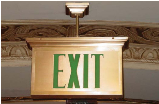
Figure 13. Careful selection, design, and location of exit signs can help preserve the historic character of significant historic spaces while still meeting code requirements. Photo: Marilyn Kaplan
