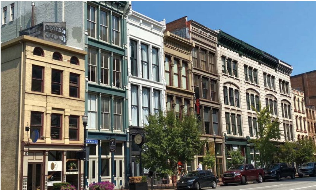
Figure 3: Some code challenges such as exiting and fire protection requirements on smaller Main Street buildings can be mitigated by using the IEBC. Photo: Marilyn Kaplan
