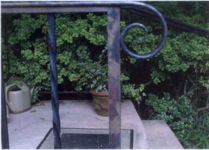
Figure 15. Metal projecting elements on a building, such as sign armatures and railings, are easily subject to rust and decay. Proper surface preparation to remove rust is essential. Special metal primers and topcoats should be used.
