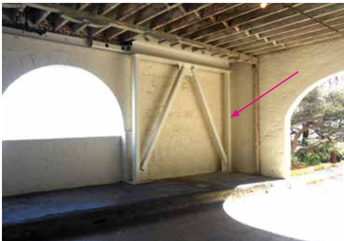
Figures 17 and 18. Careful placement of the new structural reinforcement, painted to match the surrounding building elements, if left exposed, minimizes its visual impact. New added structural elements may be left exposed when their visibility does not impair the historic character of the building. Figure 17 (left). Photo: Jason Hagin. Figure 18 (right). Photo: Architectural Resources Group.
