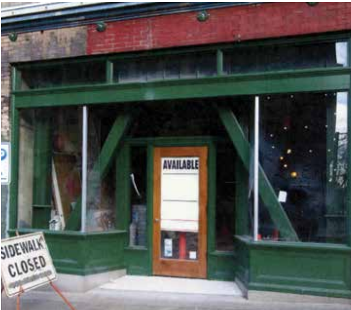
Figures 2-3. Standard approaches to seismic rehabilitation, such as adding diagonal bracing to reinforce window and storefront openings as seen in these photos, can be visually intrusive. Figure 2 (left). Figure 3 (right). Photo: Steade Craig.
