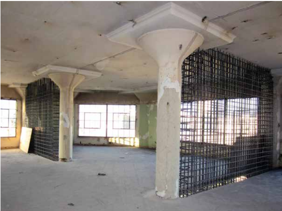
Figure 28. Steel reinforcement for the new shear walls, perpendicular to the windows, is being installed in this concrete-frame building. Photo: Robert Chattel.
