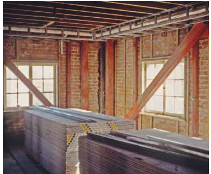
Figures 2-3. Standard approaches to seismic rehabilitation, such as adding diagonal bracing to reinforce window and storefront openings as seen in these photos, can be visually intrusive. Figure 2 (left). Figure 3 (right). Photo: Steade Craig.
