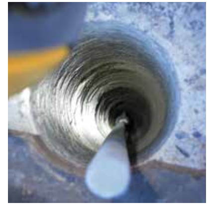
Figure 25. View of one of the center cores drilled down through the wall.
