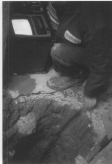
Fig. 16. Contractors specializing in building diagnostics often have video cameras or fiber optic equipment that allow the viewing of inaccessible areas. This is particularly helpful in chimney flues or subsurface drains, as shown here. In the past, these areas would need to be excavated for visual inspection. Photo: author.
