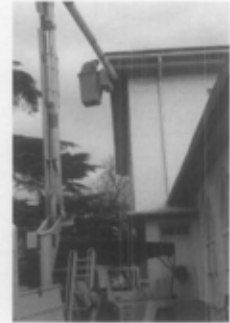
A. Inspecting the overall building on at least an annual basis will identify areas needing maintenance. A bucket lift is helpful for large buildings. Photo: author.
