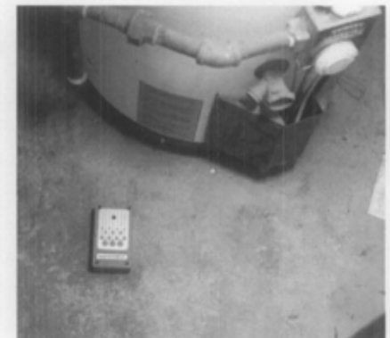
D. Protect the building from damage by maintaining equipment and using alarms, like this floor water sensor. Photo: Dell Corporation.
