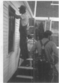
B. Repair exterior surfaces, paint, and recaulk as needed. Photo: Williamsport Preservation Training Center (WPTC), NPS.
