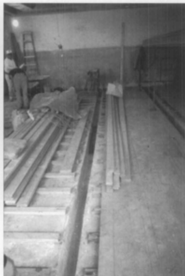
D. In a flood plain, rotted joists were replaced with a concrete slab and sleepers designed to drain water. Spaced flooring allowed drainage and room for damp wood to swell without buckling. Harper's Ferry Center, NPS.
