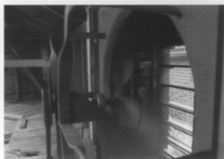
D. Install ventilating fans when additional air circulation will improve damp conditions in buildings or reduce cooling loads. Photo: Ernest A. Conrad, P. E.
