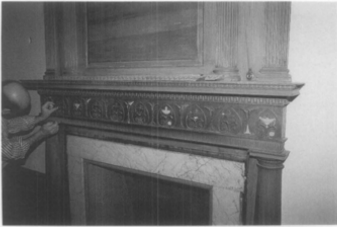
Figure 28. A conservator is replacing broken pieces of compo ornamentation on a mantel during restoration of the Nightingale-Brown House in Providence, Rhode Island. Photo: Courtesy, Irving Haynes and Associates.
