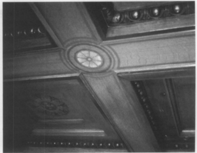
Figure 7. The coffered ceiling of the 1938 National Archives library in Washington, D.C. features egg-and-dart composition molding finished with a dark brown stain. While compo design is more often light and delicate, here, it has a bold, massive quality. Photo: Bryan Blundell.
