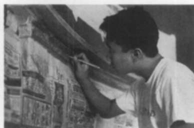
Figure 22. Careful dry scraping of a chimney piece to remove paint residue signaled the successful conclusion of a conservation project at the Octagon House, in Washington, D.C. Photo: Lonnie J. Hovey, AIA.
