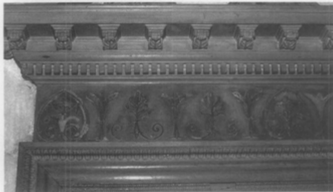
Figure 12. The Nightingale-Brown House, in Providence, Rhode Island, was built in 1792. Original composition ornament can be seen in the flat area above the door molding; matching ornament was used in the room over the mantel. Photo: Courtesy, Irving Haynes and Associates.
