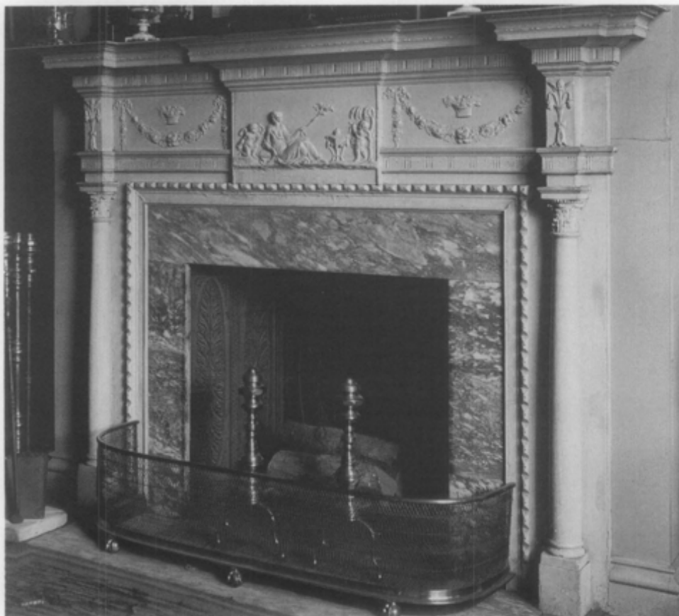
Figure 1. An American mantelpiece in the Adam style dating from the early 19th century illustrates composition ornament's reputation as a first-rate imitator of wood. Only the allegorical design, flower baskets, floral swags or festoons, flanking fleur-de-lis ornamentation and pilaster capitals are compo; the panels and simple moldings are carved wood. Photo: Courtesy, Philadelphia Museum of Art; Given by Mrs. Thurston Mason in memory of her sister, Miss Anna P. Stevenson.
