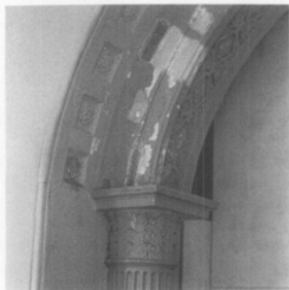
Figure 20. The Octagon House, in Washington, D.C., was constructed between 1801-1802. During recent project work, it was discovered that early repairs to the composition ornament in this doorway had been made with plaster. The plaster repairs were removed during restoration of the doorway to its original appearance. Photo: Lonnie J. Hovey, AIA.
