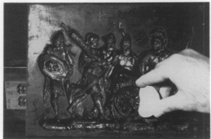
Figure 27. When a compo frieze depicting The Triumph of Mars was found to be damaged, improperly restored, and its intricate design clogged with paint, the first step was to replace a missing wheel on the chariot. Because molds depicting classical themes are part of many professional studio collections, it was possible to fabricate a new wheel from the rubber mold shown here. Photo: William Adair.
