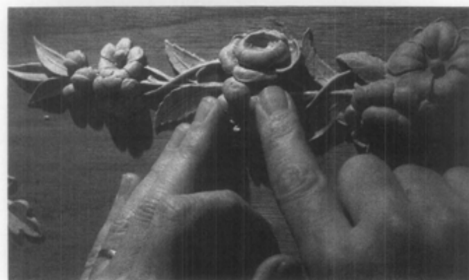
Figure 25. (a) Adhesive is being applied to this 19th century composition ornament that has de-laminated from its wood substrate; and (b) The compo fragment is held in place until the quick-setting adhesive takes hold. Photos: Jonathan Thornton .
