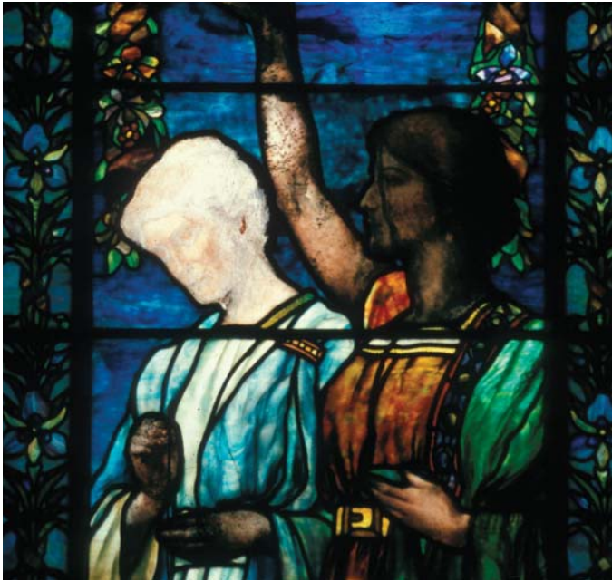
Figure 11. The face paint has failed substantially in the figure at the left. Ghost images of the feature are barely visible. Window (1903) by Edwin P. Sperry, glass by Tiffany Studios; “Old Main,” (1891-1893) Illinois Institute of Technology, Chicago. Photo: Rolf Achilles.
