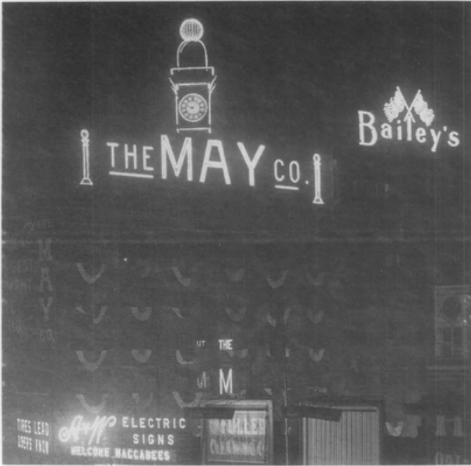
6. This view of Cleveland taken about 1910 shows how electricity transformed American cities. These dramatic and highly visible signs no doubt provided excellent advertising for "A & W Electric Signs." Its signs—at the bottom of the photograph—also proclaim the company to be the "exclusive agents" for a maker of "electric on enamel signs." Photo: Library of Congress.
