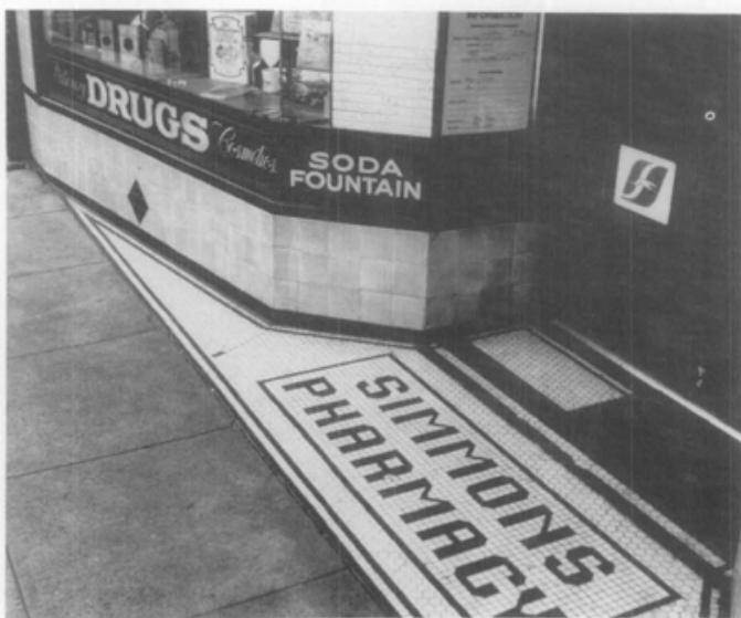
13. Historic signs were often built into a property—and often under foot. Photo: Richard Wagner, National Trust for Historic Preservation.
