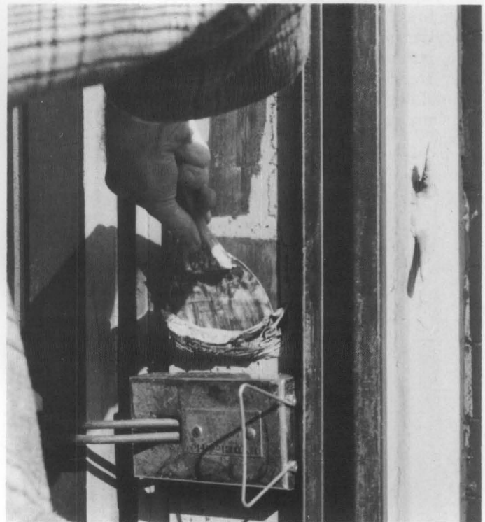
Fig. 13 The electric heat plate (with paint scraper) is particularly useful for removing paint down to bare wood on flat surfaces such as doors, window frames, and siding. After scraping, some light sanding will probably be necessary to smooth the surface prior to application of primer and top coats. Photo: David W. Look, AIA.
