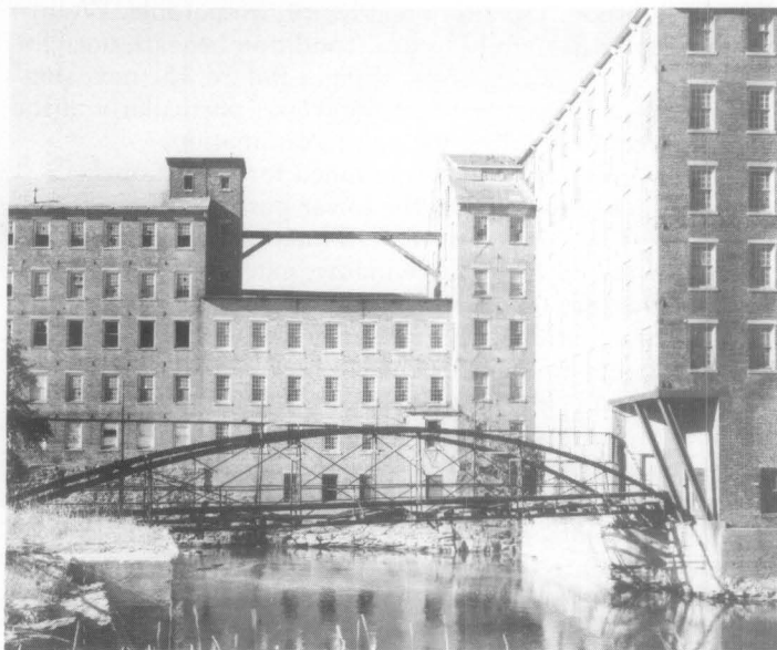
Figure 1. Windows are frequently important visual focal points, especially on simple facades such as this mill building. Replacement of the multi-pane windows here with larger panes could dramatically change the appearance of the building. The areas of missing windows convey the impression of such a change. Photo: John T. Lowe
