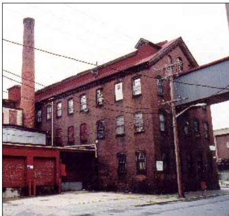
Industrial building and bridge before rehabilitation.
