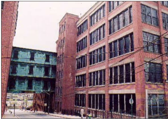
Industrial bridge before rehabilitation.
