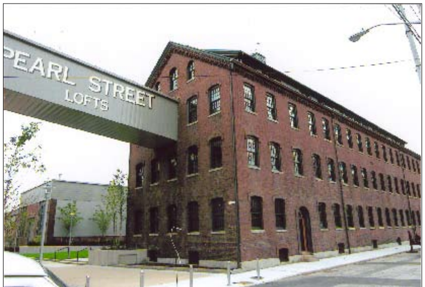
Industrial building and bridge after rehabilitation.
