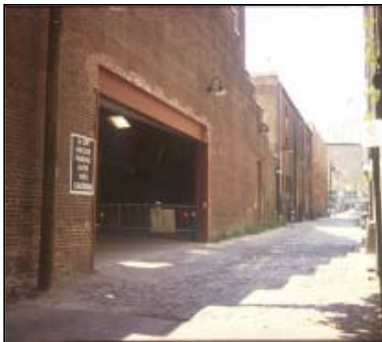
The new parking entrance is appropriately located along an alley where two smaller openings were enlarged to accommodate vehicular traffic.
