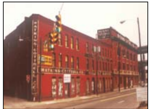
This brick warehouse complex built between 1865 and 1905 was converted to commercial and retail uses. A concealed rear structure worked well for interior parking.
