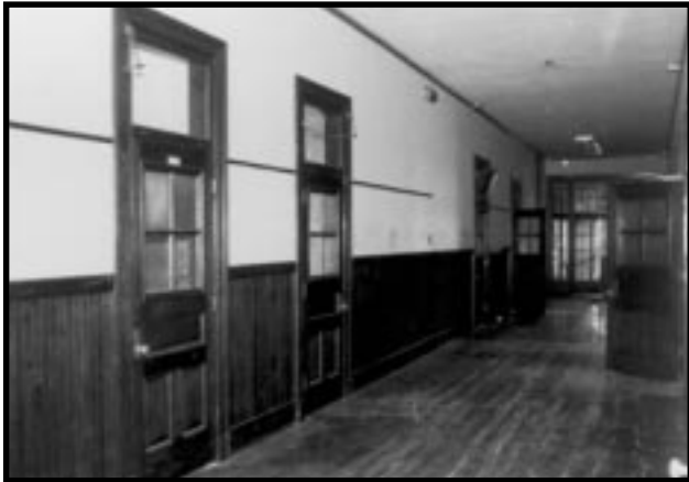
Second floor hallway prior to rehabilitation.
