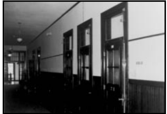
Second floor hallway after rehabilitation. Note retention of historic fabric.
