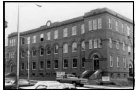
The school after rehabilitation. Windows, doors, and transoms were repaired. The building was not cleaned.
