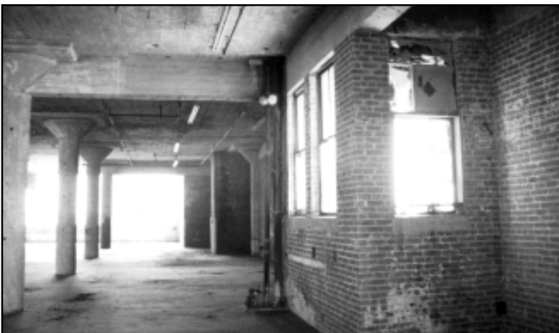
The masonry walls were historically left unfinished. Exposed brick would therefore be an appropriate treatment for the rehabilitation of this building.
