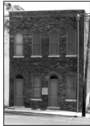
Built in 1879, this commercial/residential structure is an example of a building type where exposed brick is not an appropriate interior wall treatment.
