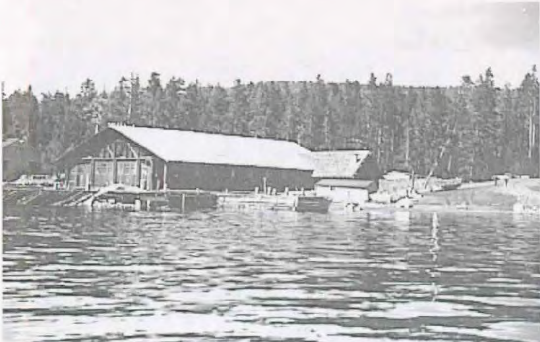
Figure 5.16. Lake boathouse (YELL Archives photo no. 61 699).
