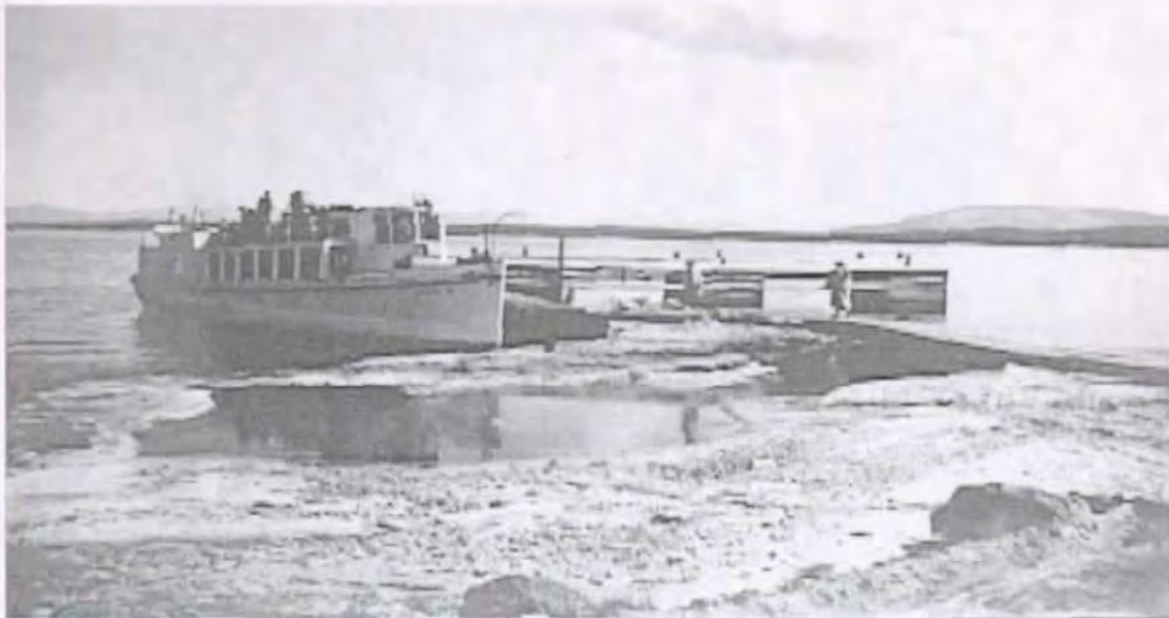
Figure 5.9. Jean D docked at West Thumb. Note the cribbing and walkway (YELL Archives photo no. 88438).
