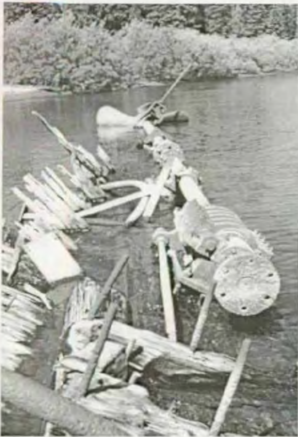
Figure 5.37. View west of E. C. Waters' propulsion system. The engine bed is in the foreground, the thrust bearing is in the middle foreground and the propeller shaft and the propeller is in the background. NPS photo by John Brooks.
