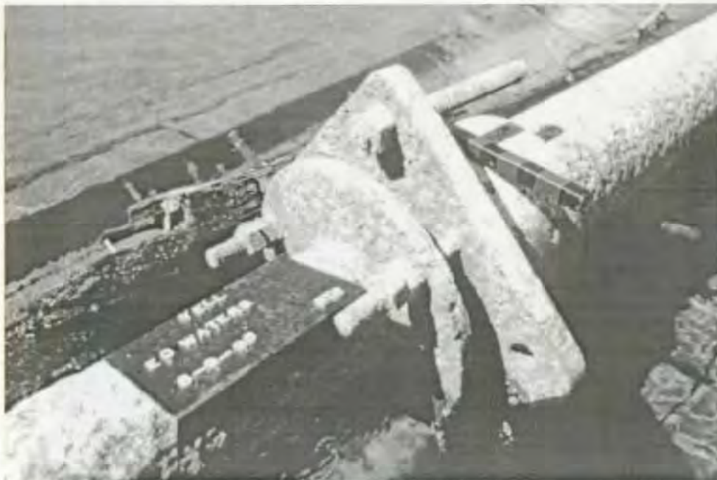
Figure 5.42. View southwest of forward end of stern tube stuffing box and gland. Note large bolt on top that secured the shaft to the stern deadwood (now missing) through which it passed. Marked section of scale = 6 inches. NPS photo by Brett Seymour.
