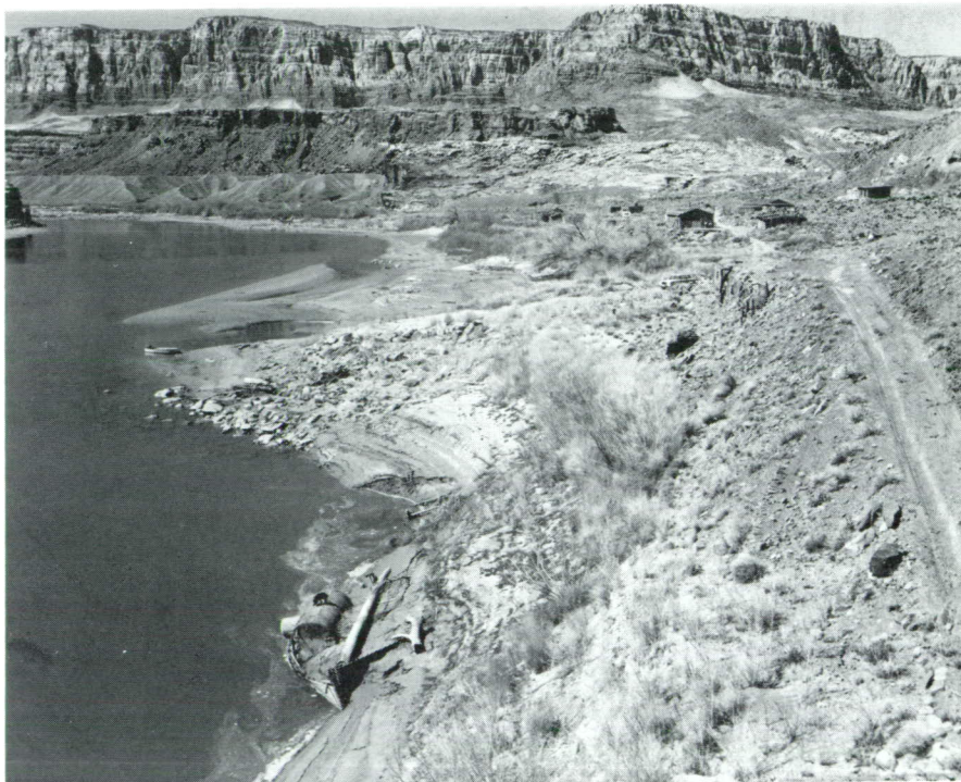
Figure 3.25. View downstream of the Spencer area as it appeared in 1963. Remains of the CHARLES H. SPENCER lay partially submerged in the foreground. The old road to the ferry is at right. Note the good condition of the USGS buildings. Photo by W. L. Rusho. Courtesy Bureau of Reclamation.
