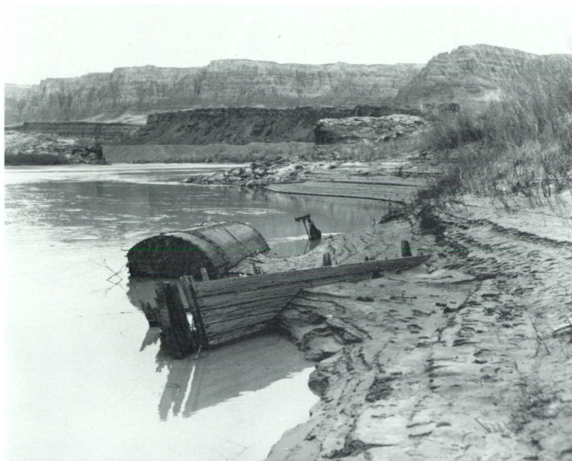
Figure 7.17 Condition of the boiler and the bilge pump in situ, March 1962. Photo by W. L. Rusho.
