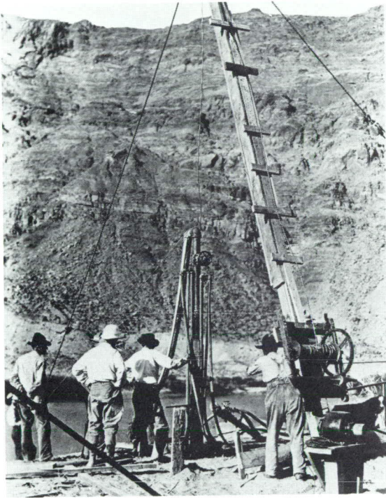
Figure 3.6. (Left) The Lovett pipe dredge in operation. C. H. Spencer (with hand on pipe) oversees nozzle withdrawal. Photo by A. H. Jones, August 1910. Courtesy W. L. Rusho.
