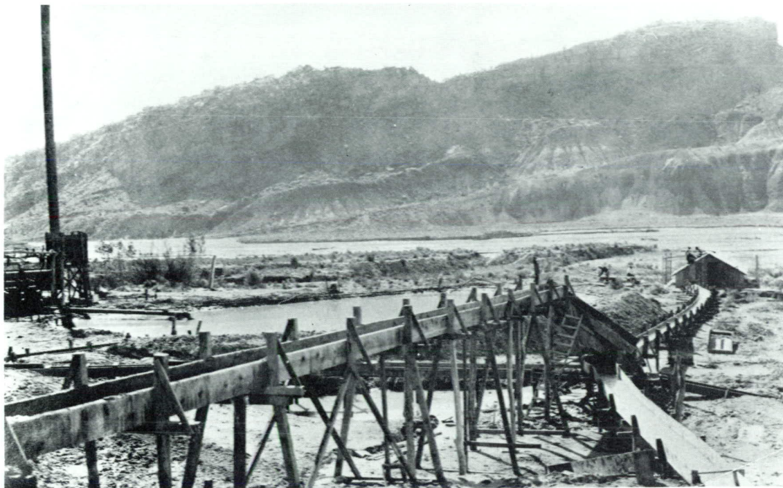
Figure 2.2. The long flume at Paria Creek, set up in late 1909 or early 1910, was used to carry the sluiced silts from the cliff to the amalgamators by the river. This arrangement was similar to the set up at Lee's Ferry. Courtesy W. L. Rusho.
