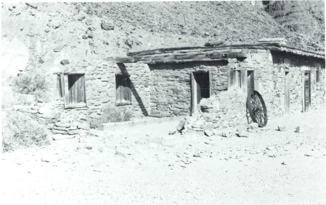
Figure 3.29. View north of Lee's Ferry Fort in 1986 showing the collapsed walls of the Spencer addition on the south end of the fort. Note the steel wheel from the boiler. Photo by J. Bradford.
