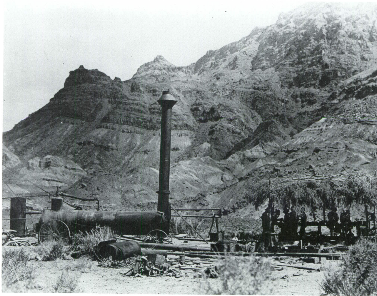
Figure 3.5. Boiler used to operate a small water pump and air compressor connected to the Lovett pipe dredge. The nozzle of the dredge can be seen extending out of the left side of the ramada. Photo by A. H. Jones, August 1910. Courtesy W. L. Rusho.
