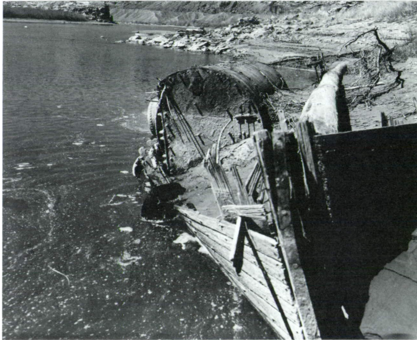
Figure 6.5 The bow of CHARLES H. SPENCER had deteriorated considerably by 1963. The small hand pump is still in place, however the boiler had rolled over onto the starboard side. Photo by W. L. Rusho.
