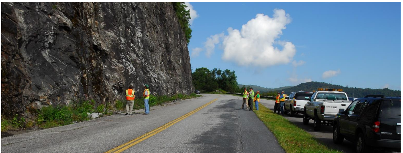
NPS staff conducting a Road Safety Audit on the Blue Ridge Parkway
