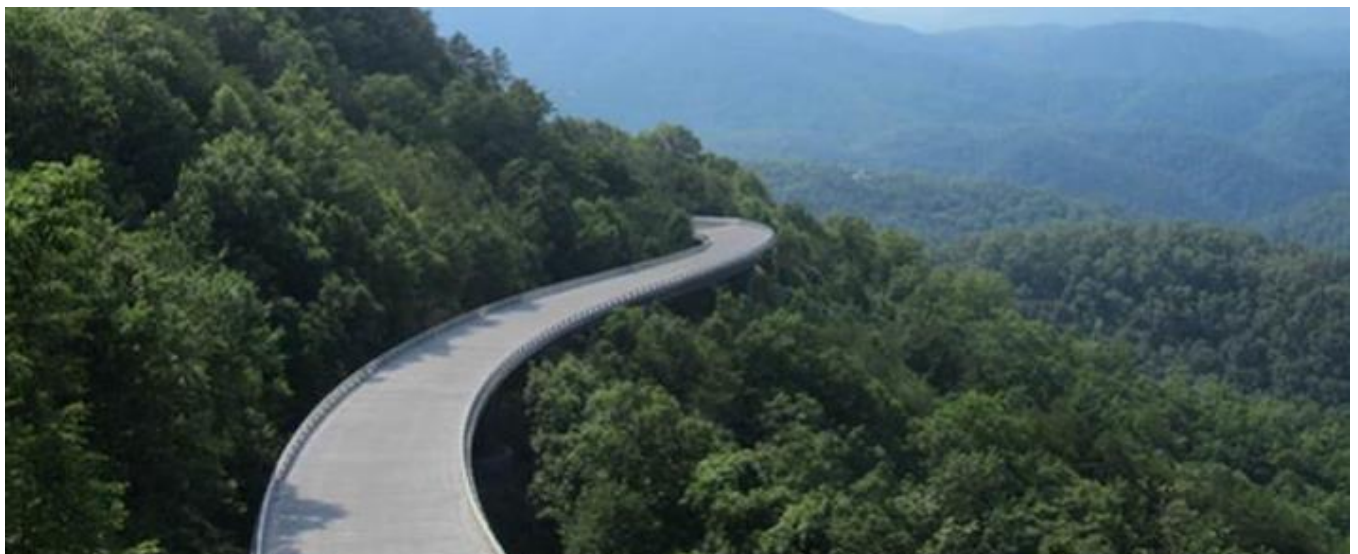
One of a series of bridges that make up part of the “missing link” of the Foothills Parkway at Great Smoky Mountains National Park
