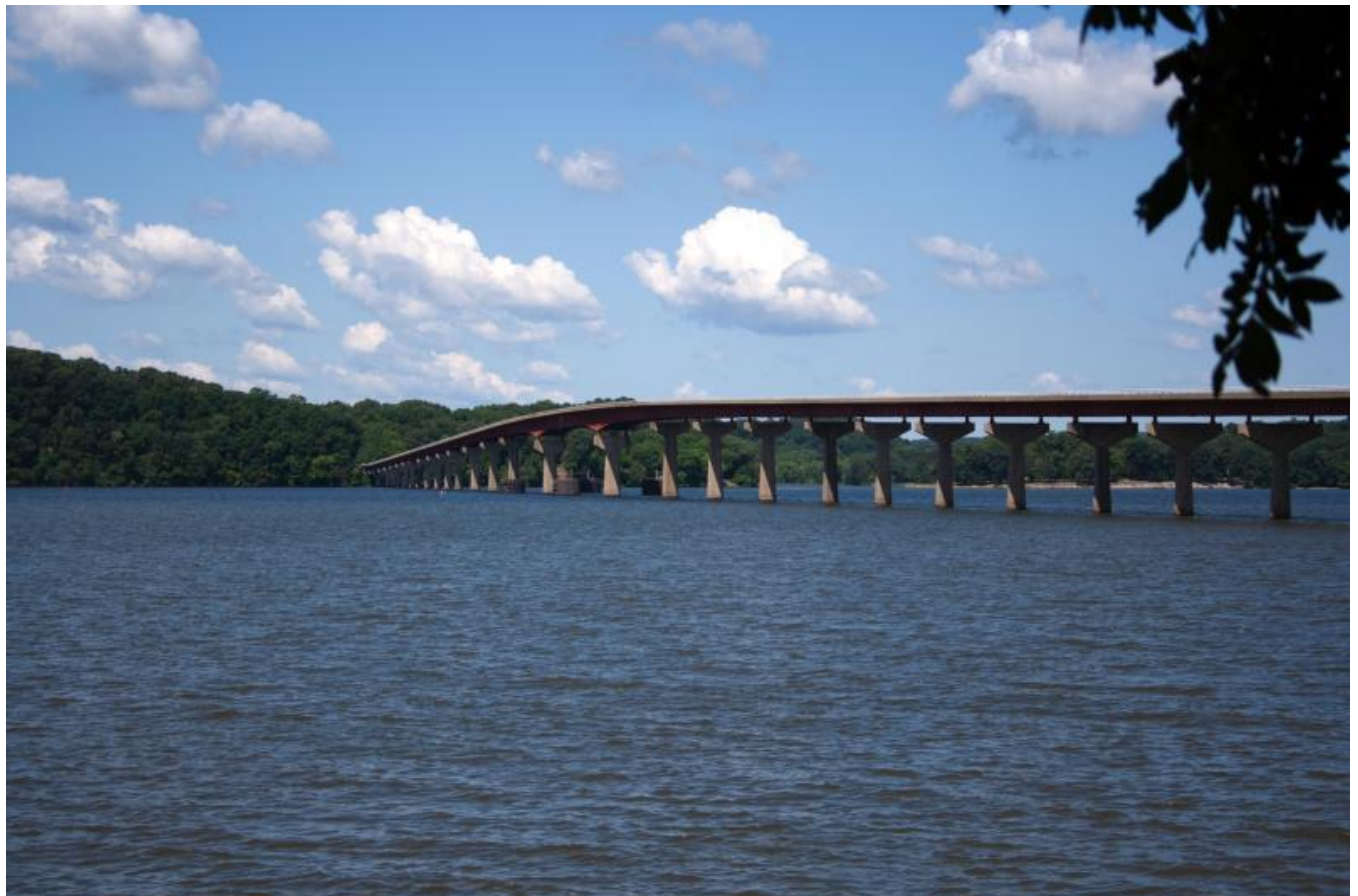
John Coffee Memorial Bridge on the Natchez Trace Parkway
