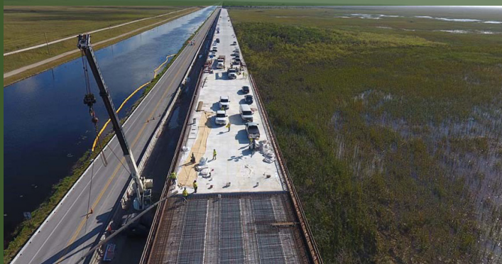
Tamiami Trail Bridge at Everglades National Park
