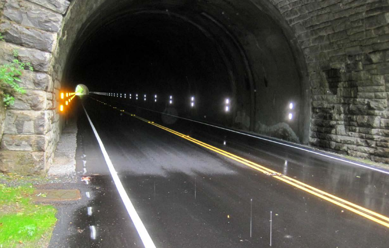
The Tanbark Ridge Tunnel at Blue Ridge National Park.
