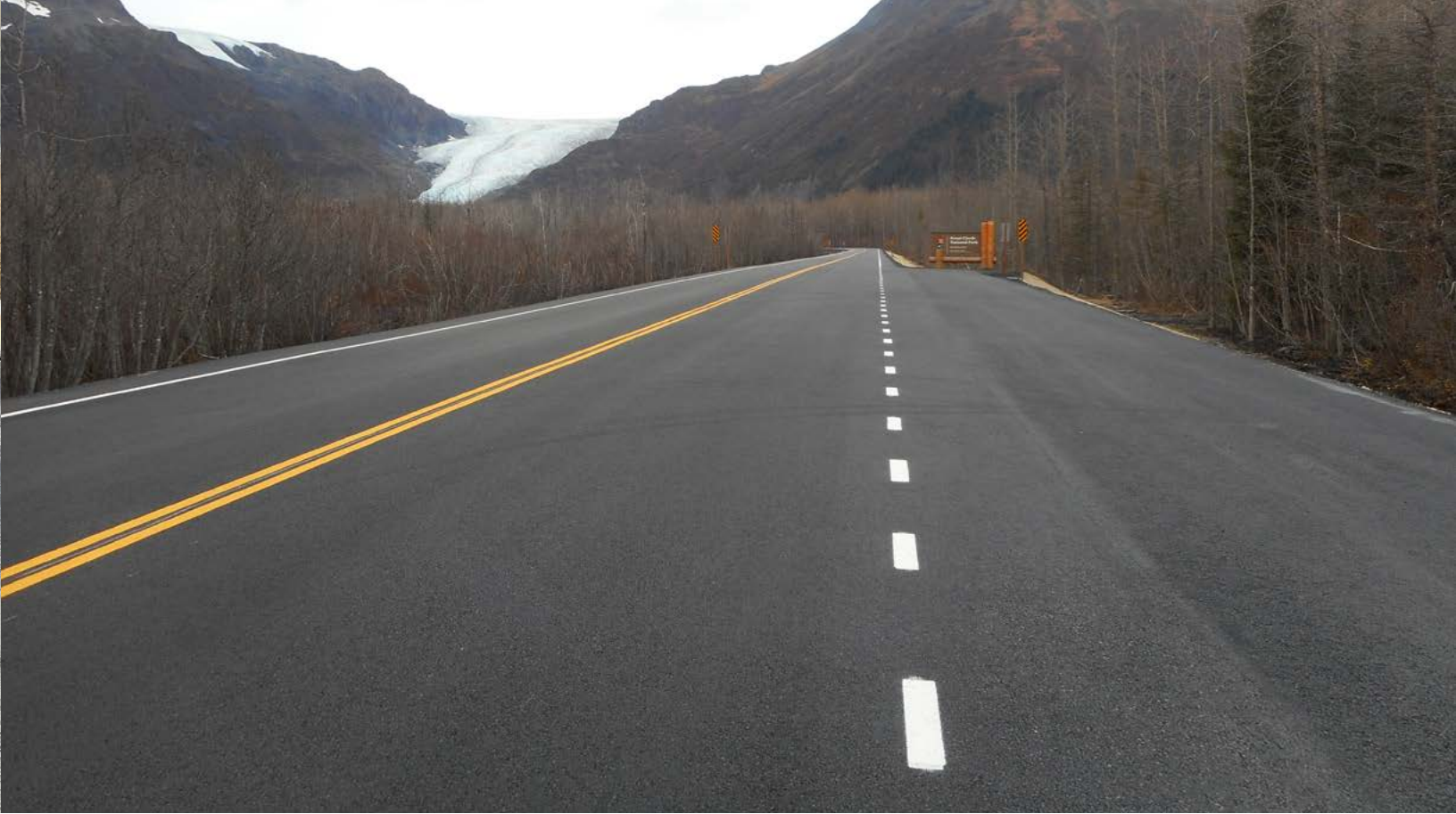
Completed resurfacing work on Glacier Road in Kenai Fjords National Park.
