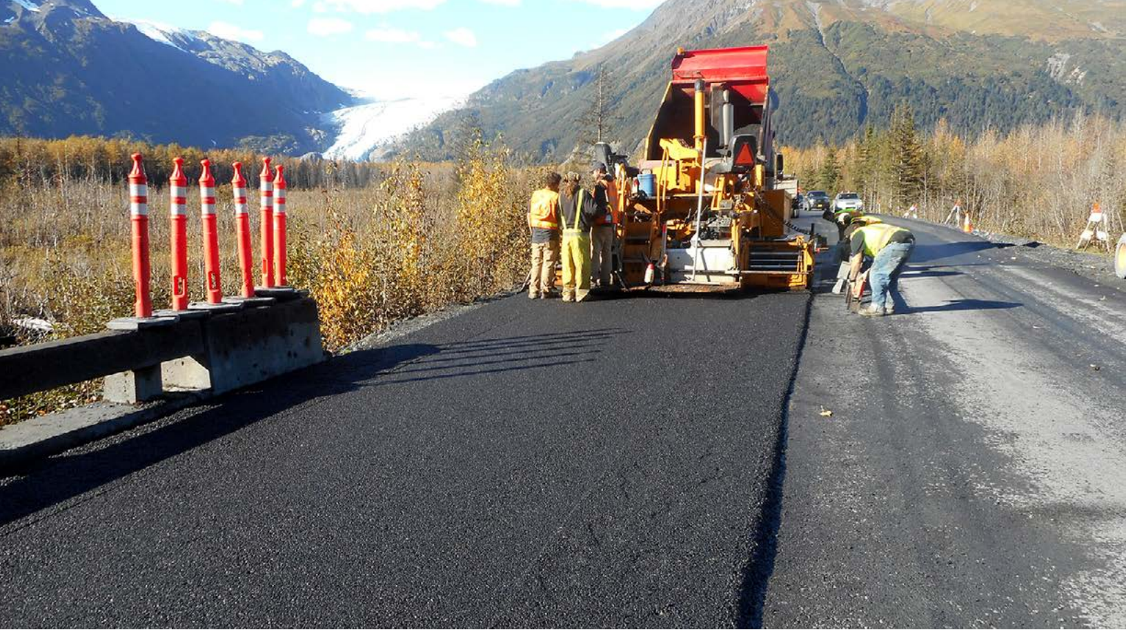
Resurfacing work on Glacier Road in Kenai Fjords National Park.
