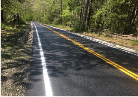
Completed road and drainage rehabilitation at Delaware Water Gap National Recreation Area. (NPS Photo)
