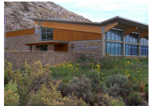
Before and after revegetation outside the visitor center at Dinosaur National Monument. (Photo:NPS)
