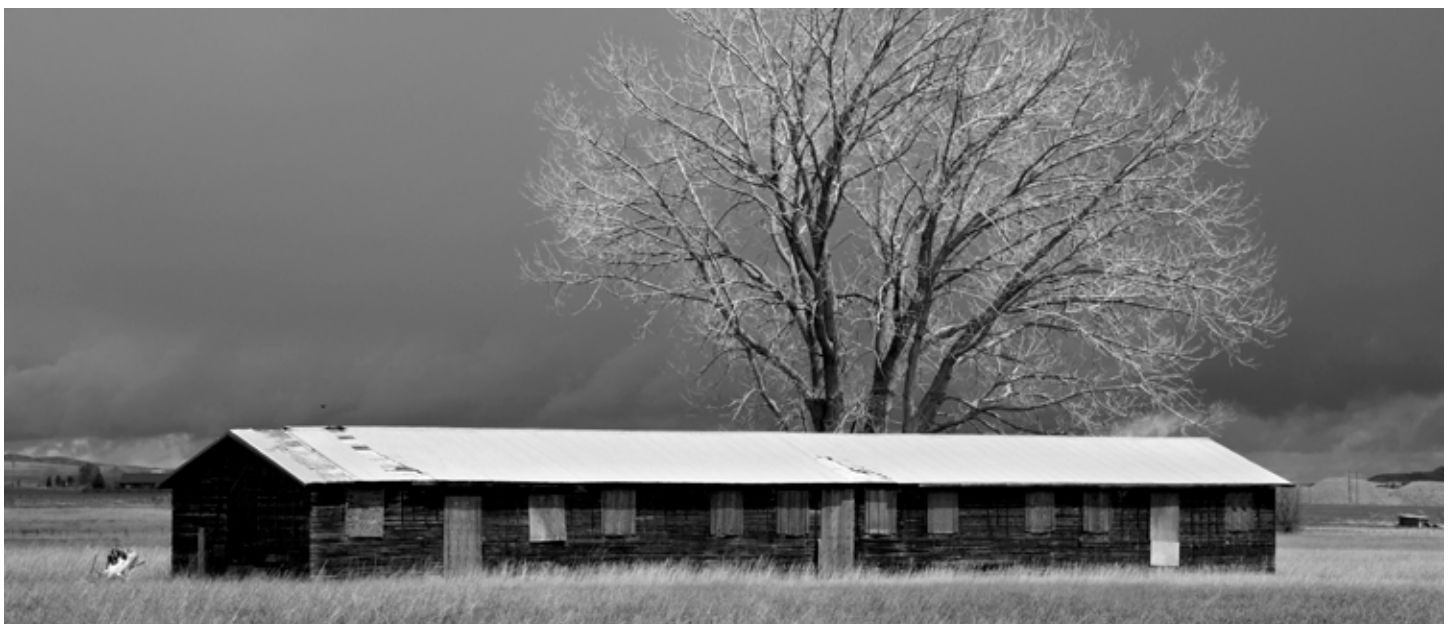
A barracks building found outside of Cody, Wyoming, was moved from its original location at the historic Heart Mountain incarceration site. Photo by Stan Honda, courtesy of Moving Walls project.
