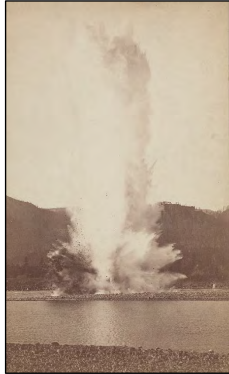
Figure 47. The US Army Corps of Engineers blasted the riverbed in preparation for constructing the Cascade Locks and Canal. Photograph by Carleton E. Watkins, 1883.
