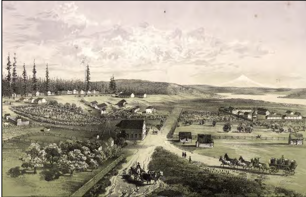
Figure 44. Gustavas Sohon completed this lithograph of Fort Vancouver in 1854. It depicts the period when the US Army and the HBC shared the area. The HBC buildings are on the right, while the more recent US military buildings are on the left, up the hill from the original fort.
