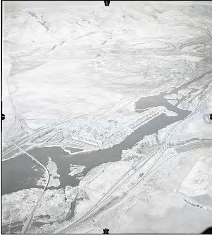
Figure 54. Dalles Dam under construction in 1955. The Long Narrows (Dalles Rapids) and Big Eddy are on the right-hand side of the image. The Short Narrows (Little Dalles Rapids) and Celilo Falls are upstream, or to the right, of what is visible here.
