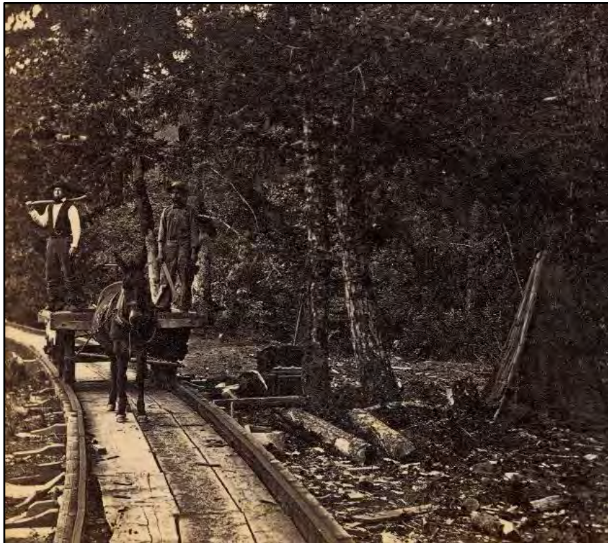
Figure 31. The mule-powered tramway pictured here is the Oregon Portage Railroad, on the Oregon side, which at one point had a small steam locomotive (“The Oregon Pony”), but after its retirement, the operator of the Eagle Creek Sawmill used mules to carry cars over the wooden railroad. This system is similar to what Bradford operated on the Washington side of the portage starting in 1851. Stereoview by Carleton E. Watkins, 1867.
