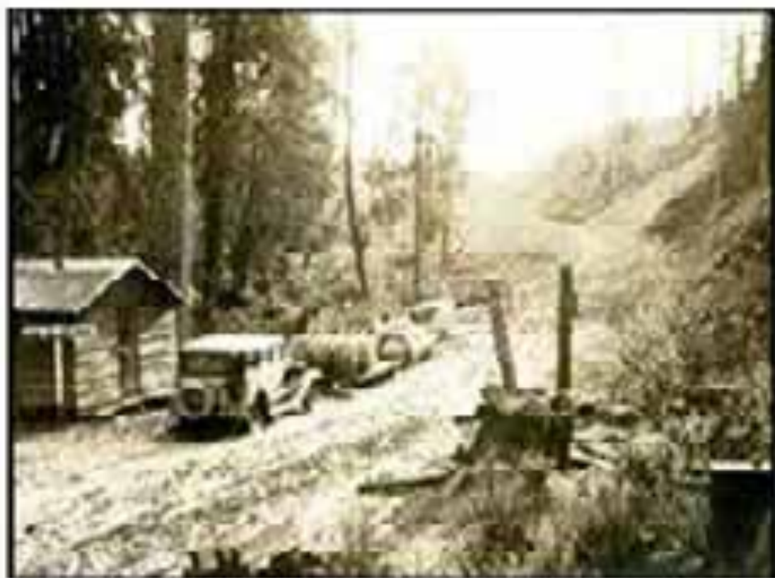
"End of the Road" to Queen's Bridge construction. Courtesy Jim Hestings.
