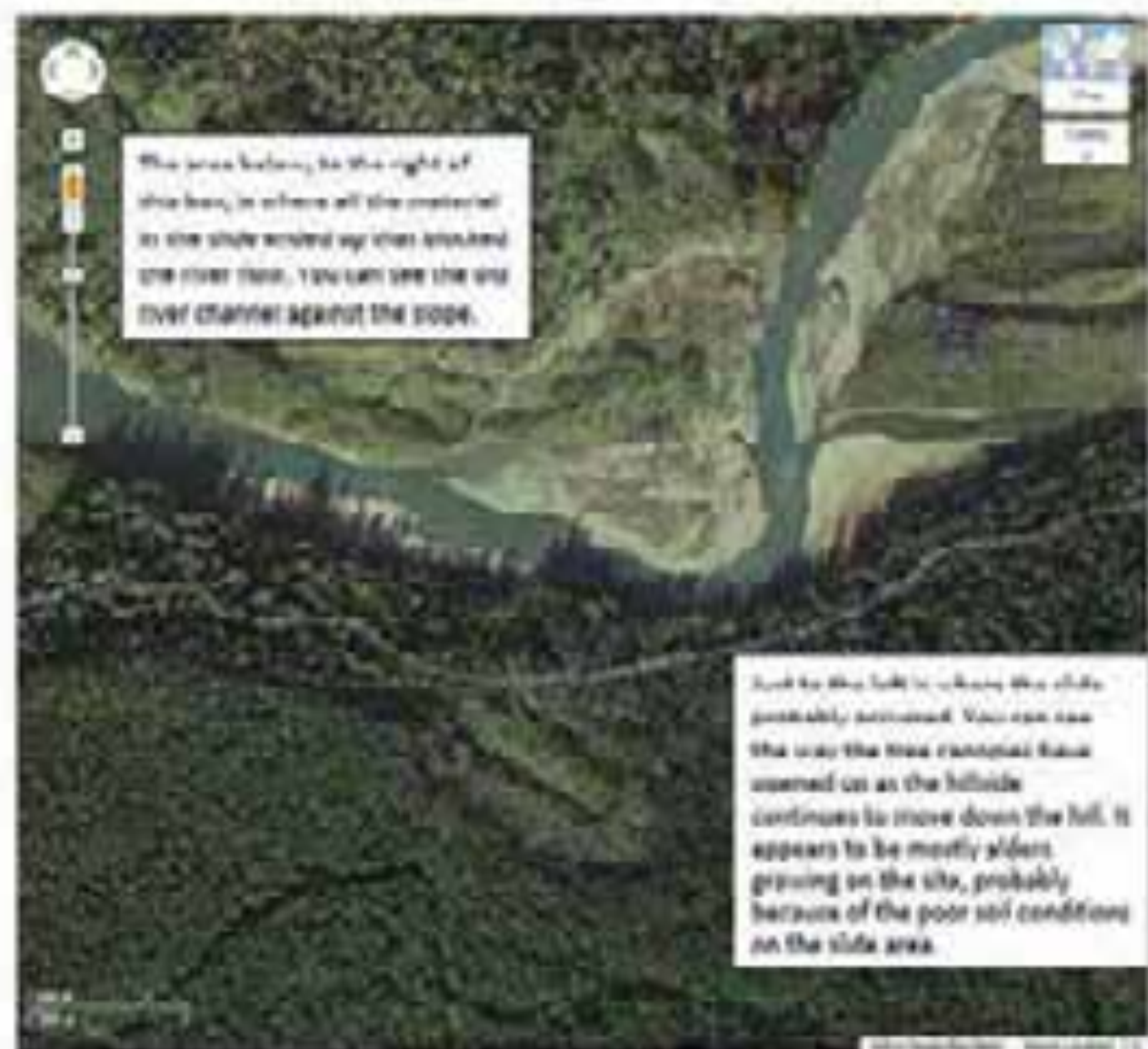
The second slide that blocks the Quavets road is to the left of this image.
