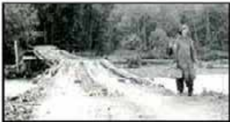
This could be the May's Doubtless bridge, circa 1910s, as it was near the Doubt and this image came from the May's photo album. The bridge would probably have been rebuilt with cement. Courtesy Joanna Crindall.
