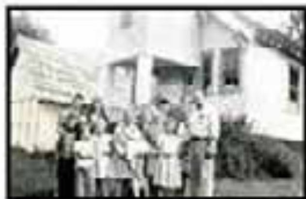
THIS IS THE SAME BUILDING IN LATER YEARS. COURTESY JIM NORTROP.
