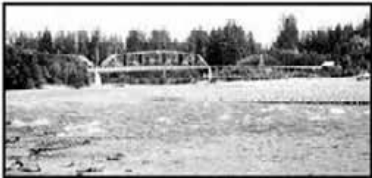
Queets River Bridge. Courtesy Joanne Grindstaff.
