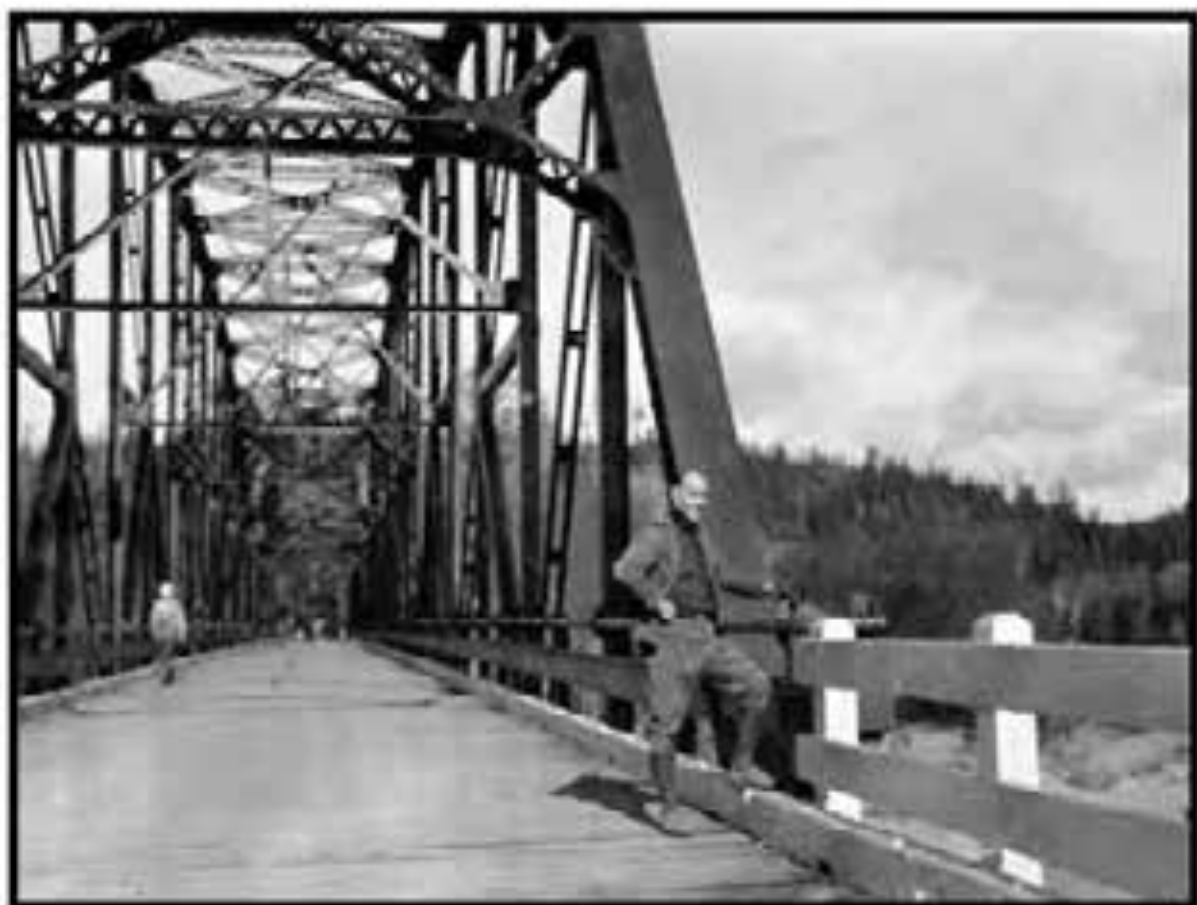
George Northup, Queets-Clearwater (county) bridge at Harlow Creek, built after state highway bridge.
