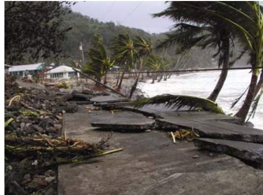
Damage to Onenoa in 2004 (Cyclone Heta).
